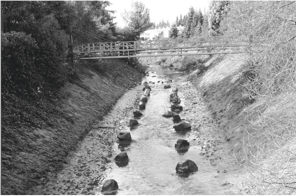
FIGURE 2.7 The Santa Rosa Creek project located in downtown Santa Rosa, Sonoma County, is an example of a single-purpose flood control project constructed in the 1960s.
