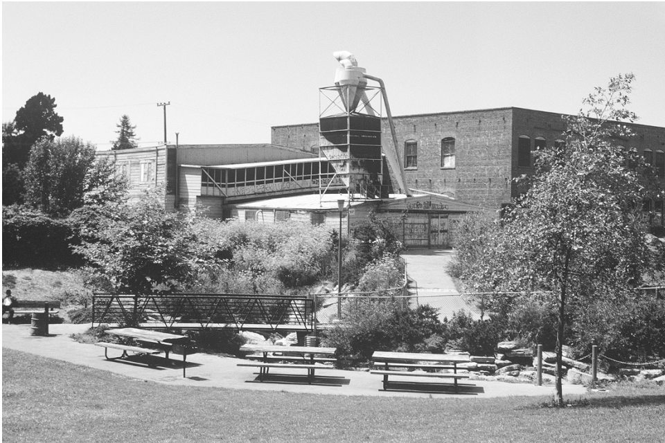
FIGURE 3.7 Strawberry Creek Park now supports offices and a café in the restored industrial building located on the creek.
