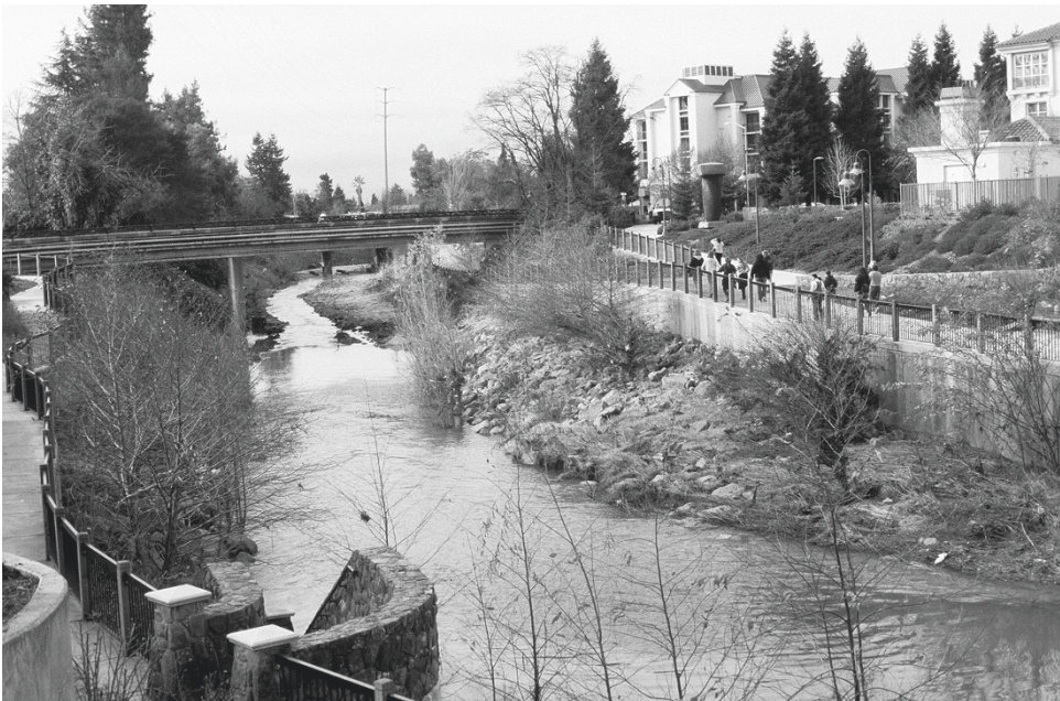
FIGURE 2.9 Restoration of ecological function to Santa Rosa Creek did not compromise the flood risk reduction objective. This photo shows the channel containing the large San Francisco north bay flood of 2005–2006.
