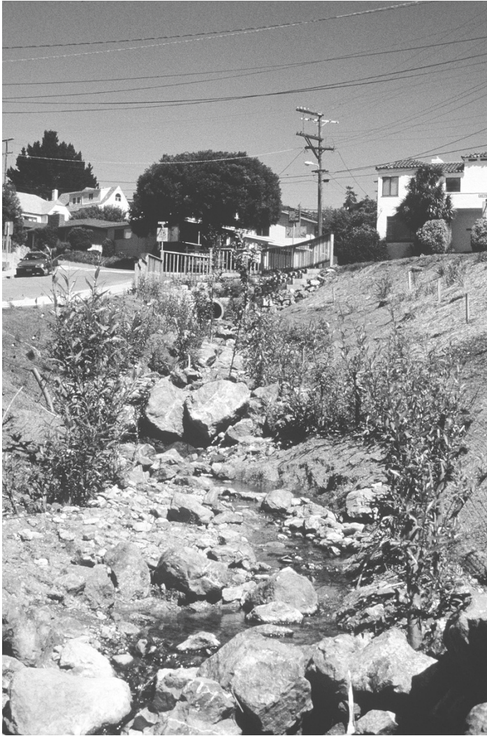
FIGURE 3.40 Transport and re-sorting of the mobile rock and cobbles by flood in early January 1997 began to rearrange the steps and pools of Baxter Creek.
