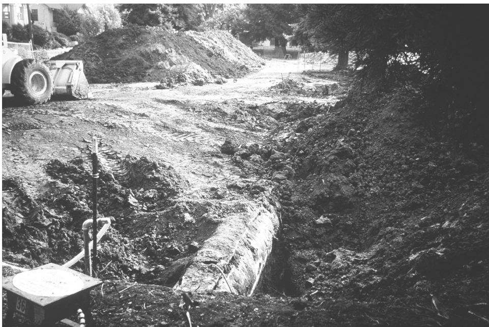
FIGURE 3.19 The Blackberry Creek culvert was excavated and cut.
