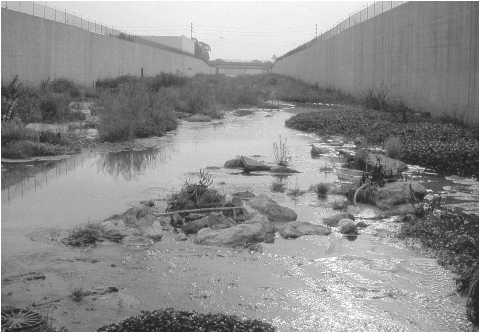
FIGURE 1.2 Coyote Creek in the San Gabriel watershed, Los Angeles County, is recovering ecological functions within a rectangular, concrete flood control channel through sediment transport, deposition, and recovery of riparian vegetation.
