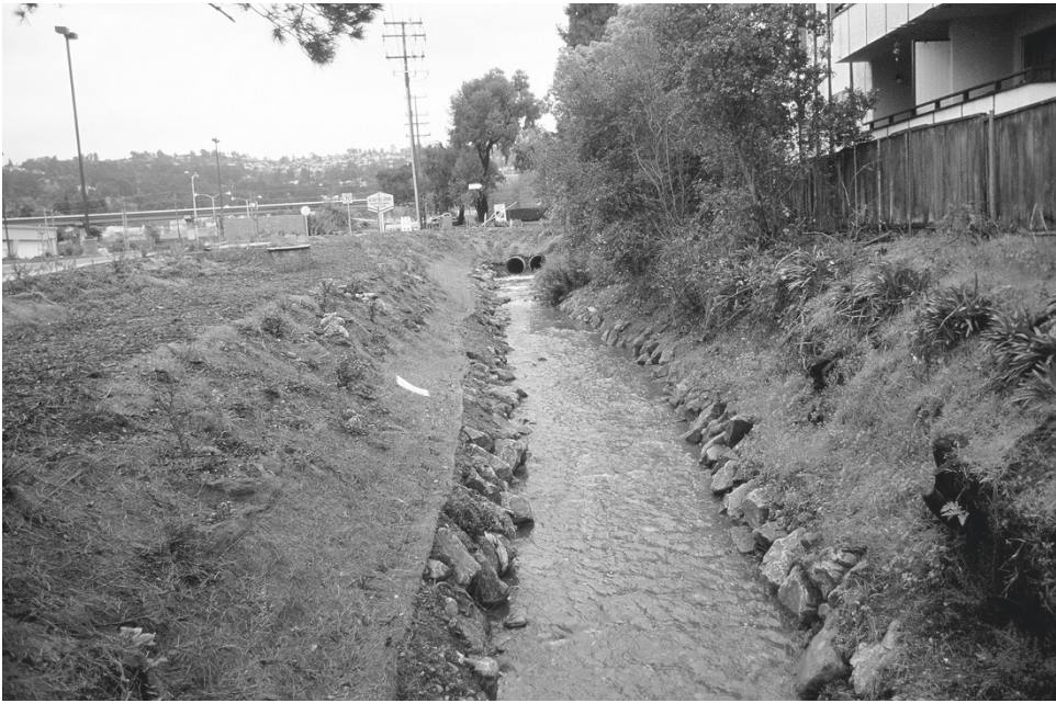
FIGURE 2.10 The Cerrito Creek Project in El Cerrito represents an enhanced, controlled channel with streamside gardening and was completed between 2000 and 2002.
