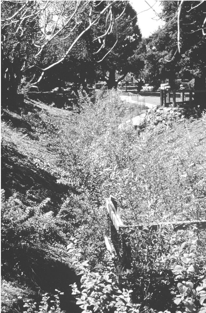
FIGURE 3.26 By the fall of 1996, one year after daylighting, the Blackberry Creek channel had a complete cover of vegetation.
