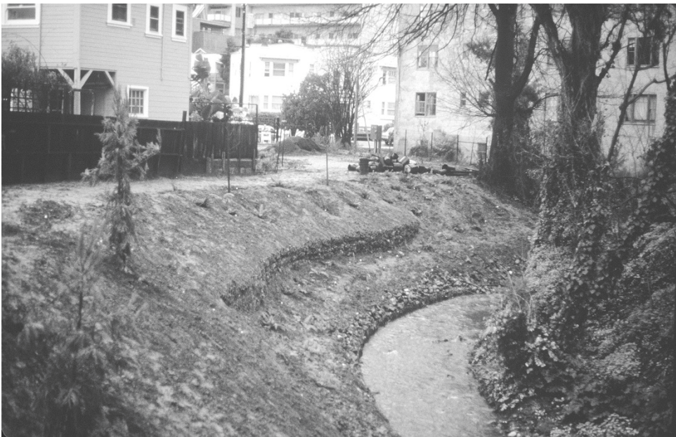
FIGURE 3.12 Plants were set into the gabion-soil medium.
