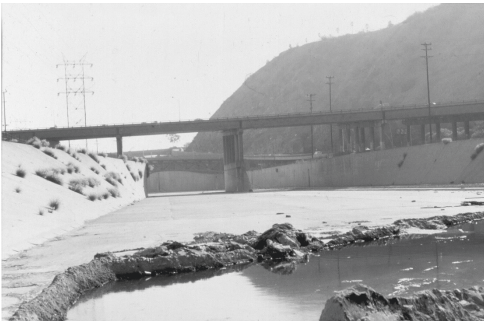
FIGURE 1.5 Nature bats last, forming a meander through the concrete bottom of the Los Angeles flood control channel.
