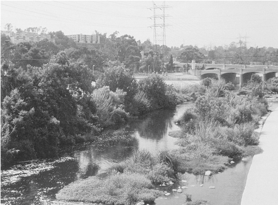
FIGURE 1.4 The Los Angeles River at “Frog Town,” Los Angeles, supports birds and aquatic habitat for amphibians in a dirt-bottom flood control channel at the 101 Freeway. Credit: Los Angeles Department of Water and Power.
