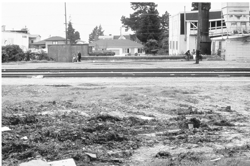
FIGURE 3.2 The Strawberry Creek site before the project was an abandoned railroad corridor and industrial woodworking building. Photo credit: Gary Mason of Wolfe Mason Associates.
