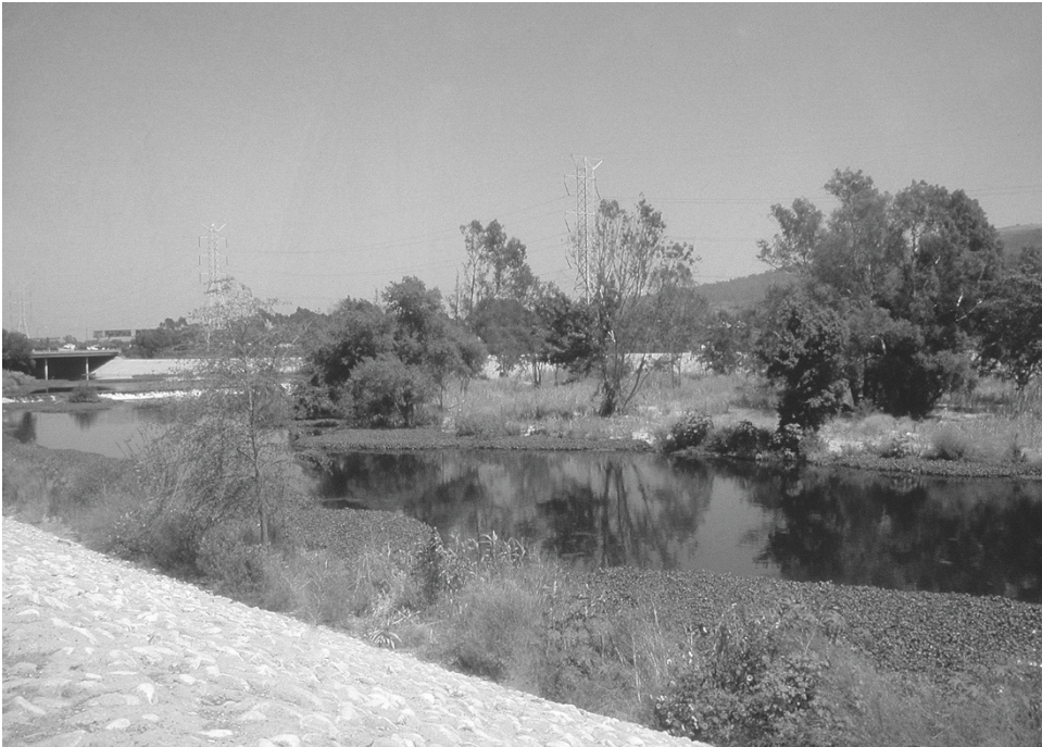
FIGURE 1.1 The North Fork Los Angeles River is re-forming in a dirt-bottom flood control channel at Glendale Narrows, Los Angeles.
