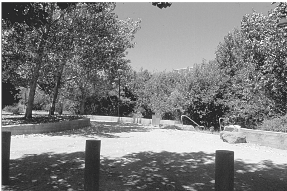
FIGURE 3.56 Project construction at Baxter Creek transformed derelict space (above) into a gateway to El Cerrito (above, opposite page), featuring creek restoration, a regional trail, and public congregation areas. Credit: Chris Benton.
