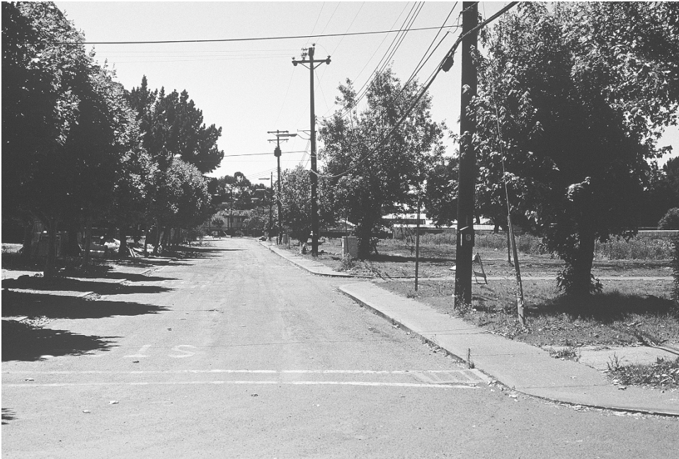
FIGURE 3.59 Before the restoration project, Village Creek flowed in an underground culvert immediately south of Riley Street.
