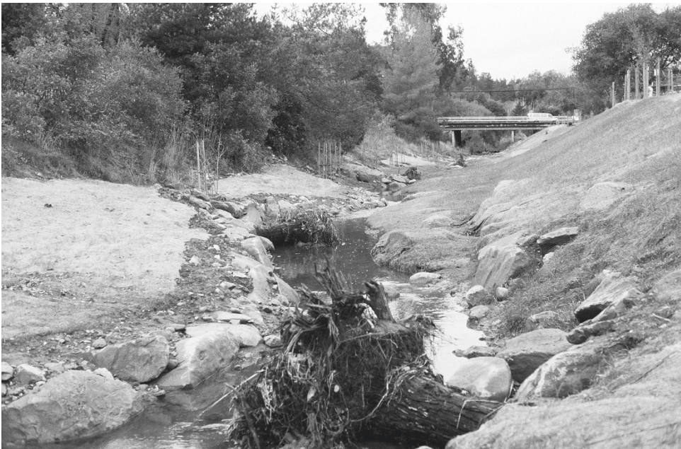
FIGURE 2.11 The 1999 Brush Creek project in the Santa Rosa area represents an enhanced-controlled channel, locking in the channel with large boulders and adding landscaping trees that do not perform ecological functions such as temperature control for the stream system.
