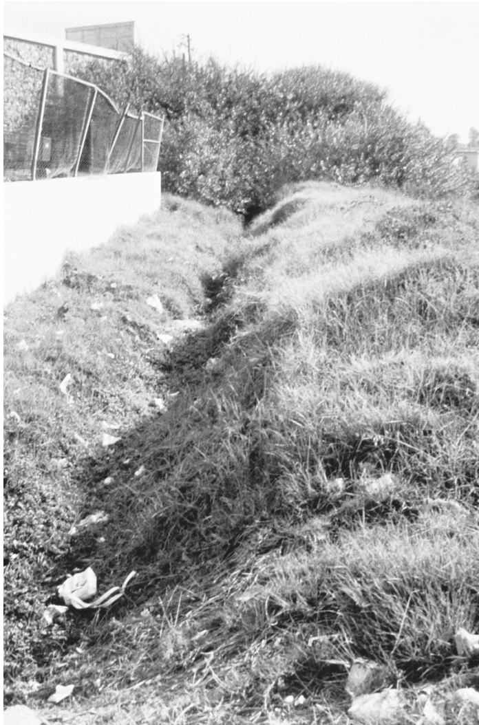
FIGURE 3.55 Before it was restored as part of a new urban greenscape, Baxter Creek was a ditch in an abandoned railway right-of-way located on a major commercial route.
