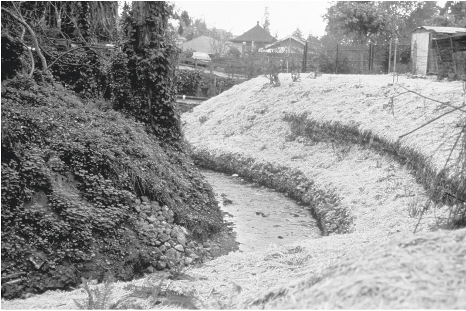
FIGURE 3.11 Straw erosion control was used to stabilize the final grading.
