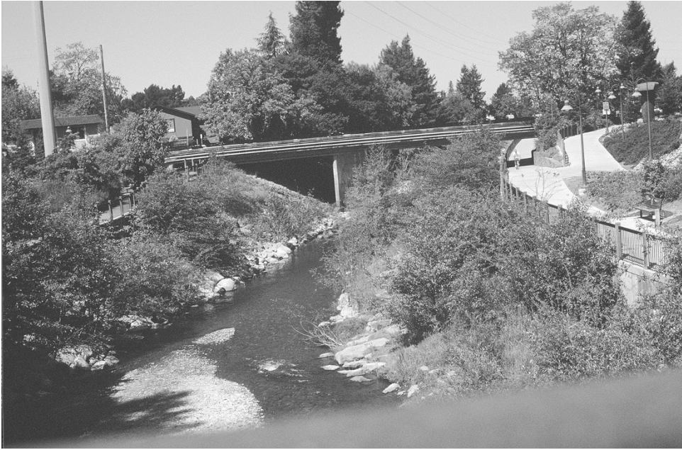
FIGURE 2.8 Removing the concrete bottom of the Santa Rosa flood control channel in 1999–2000 allowed the return of a limited functioning riparian corridor, channel sediment transport and deposition, a channel-floodplain connection, and anadromous fish passage.
