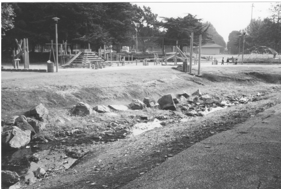
FIGURE 3.48 In 1999, before the project, Baxter Creek in Booker T. Anderson Park was a bare dirt channel with failed concrete (top) and rock riprap (bottom) banks. Photo credit: Lisa Owens Viani.
