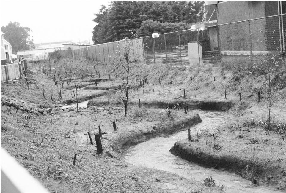
FIGURE 3.62 As part of the Village Creek project, installation of willow posts was the primary strategy for providing an inexpensive, stable, and shaded channel.
