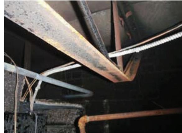
Oxidized and melted metal decking
