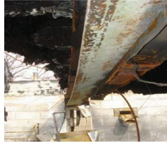
Distorted steel truss
