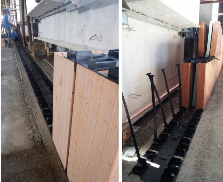
Fig. 8 Two phases of the assemblage of the PlastiBloc ® system. In evidence, at right , the plastic strips
