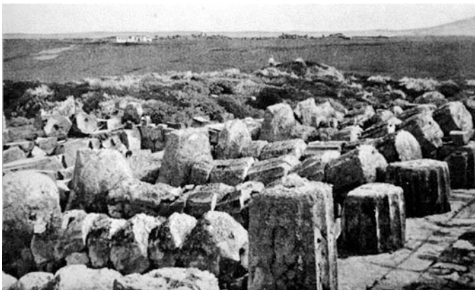
Fig. 2 The northern colonnade of Temple C (Selinunte), which collapsed as a consequence of an earthquake occurring between the 4th and the 6th centuries AD, with the characteristic domino-style arrangement of its drums (Hulot and Fougères 1910; Bottari et al. 2009)
