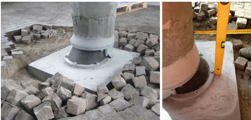
Fig. 13 Isolator device with its locking system. The isolator is deformed to its design displacement
