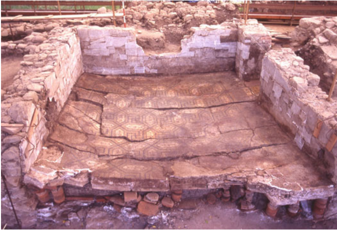
Fig. 6 Capo d'Orlando. Photo of room 4 of the Roman villa, showing the cracks across the floor in an E–W direction and in the internal walls of the room (after Bottari et al. 2008)
