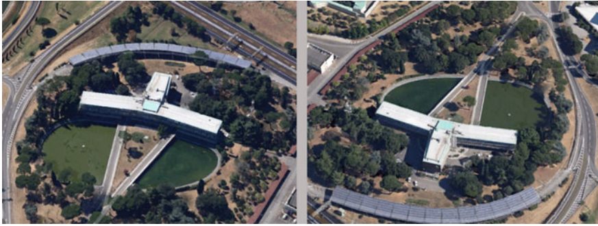
Fig. 1 Aerial view of the building
