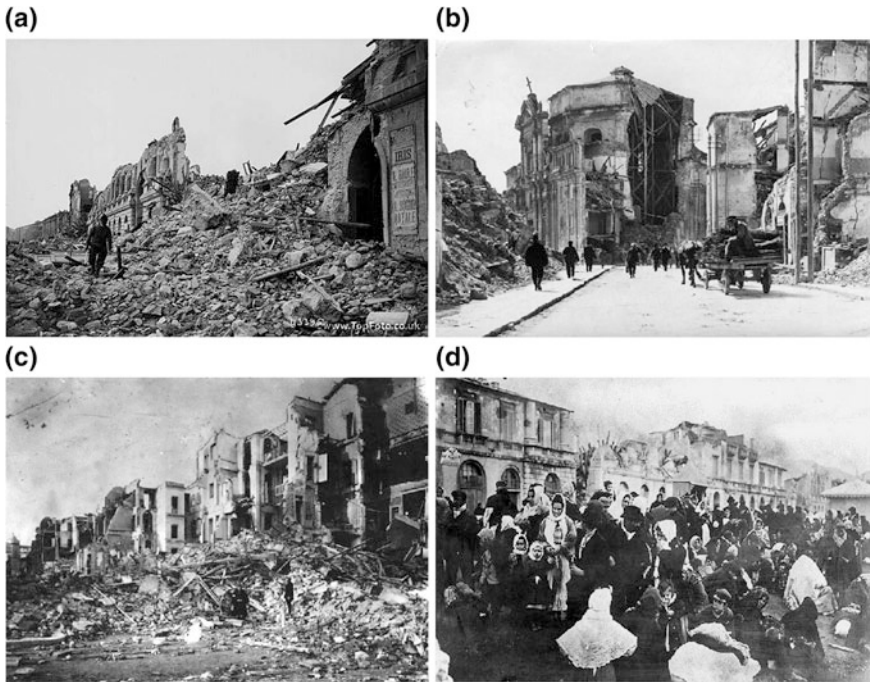
Fig. 3 a Structural damage of masonry buildings in Messina ( raafyawan.wordpress.com ). b Structural damage of masonry buildings in Messina ( www.telegraph.co.uk ). c Structural damage of masonry buildings in Messina. d Refugees awaiting transportation at Messina ( www.ibiblio.org )
