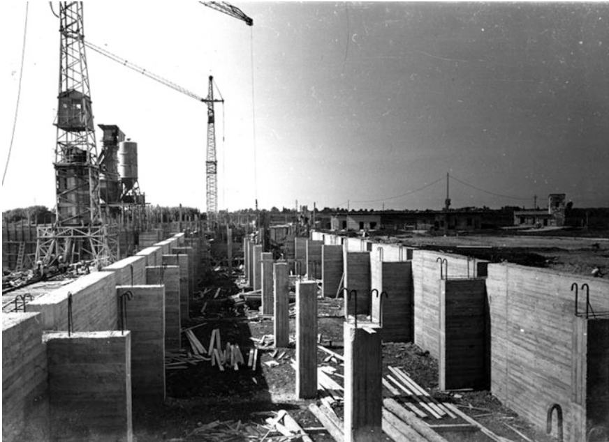
Fig. 7 Shows an archive picture taken during construction of the basement area; the reinforced concrete columns that today support the isolating devices are clearly visible
