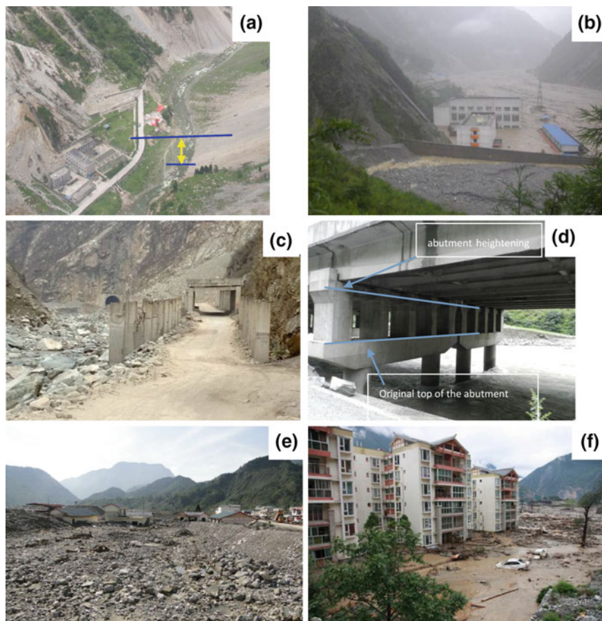
Fig. 5 a The river bed near Xiaomuling power station on 14th, May, 2008. b Rise of the river bed at the Xiaomuling power station on 9th, July, 2013. c Abandoned shed-tunnel along Yuzixi River due to the rise of the river bed. d Redesign of bridge Pier. e New houses buried by a debris flow in Qingping. f Apartment building in the outflow area destroyed by debris flows
