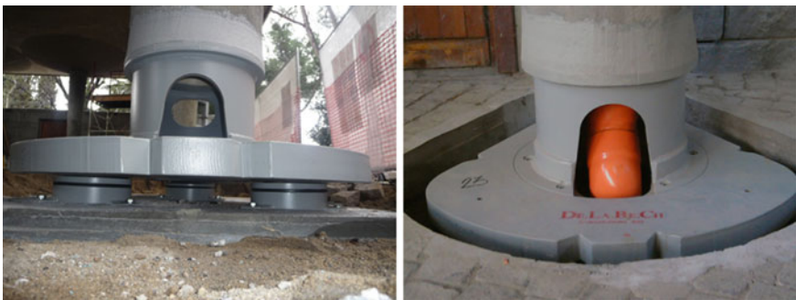
Fig. 11 Left support points at the base of “tripods”. Right the internal flexible joint
