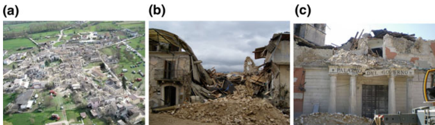
Fig. 3 Onna city after the April 6, 2009 seismic event struck (a, b); L'Aquila city (c)
