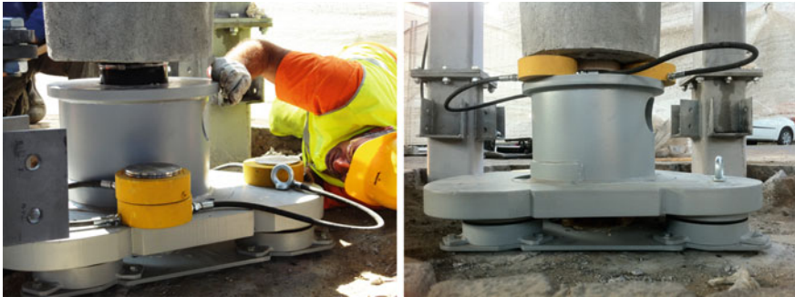
Fig. 12 A “tripod” during the installation phases
