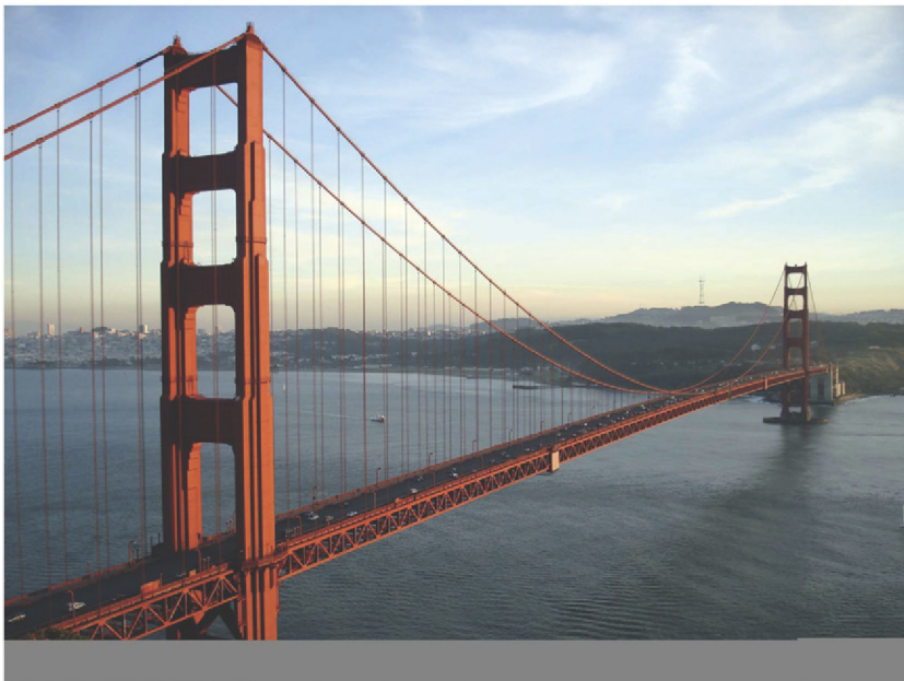
FIGURE 7.3 Golden Gate Bridge, San Francisco, California. (Source: Rich Niewiowski, Jr., http://en.wikipedia.org/wiki/File:GoldenGateBridge-001.jpg .)
