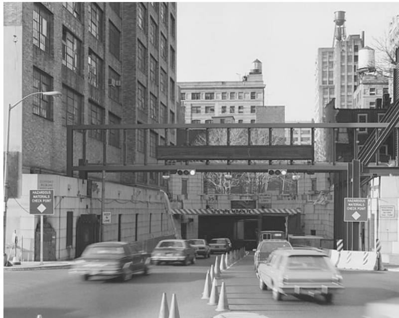
FIGURE 3.5 Entrance to the Holland Tunnel in New York City. (Source: National Park Service, http://en.wikipedia.org/wiki/File:Haer_hollandtunnel.jpg .)
