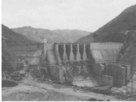
PHOTO 1. Dachaoshan Dam, the second dam on the Mekong River's mainstream (February 2003 photo courtesy of Mekong Watch)
