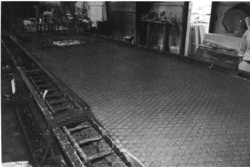
Fig. 7.3 A mixed metal oxide CP anode being cast into a newly constructed precast reinforced concrete element. These elements were used to form the pre-cast deck of a road bridge at Hauteville-sur-Fier, France.
