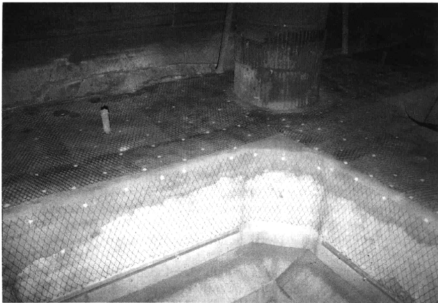
Fig. 7.1 Kwai Chung Jetty, Kowloon, Hong Kong. A double layer of anode mesh can be seen fastened to the concrete surface to provide a locally increased CP current. This increased current requirement is due to the greater embedded steel surface of the steel piles.
