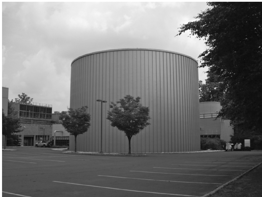
Figure 8–10 Outdoor chilled water storage tank. Asif Syed
