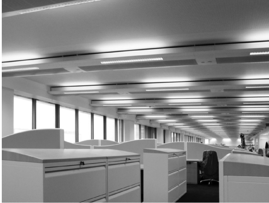
Figure 4–7 Multiservice chilled beam (without ceilings). TROX Technik
