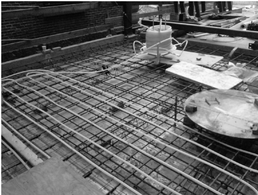
Figure 2–3 PEX tubing. Picture by J. Macaluso
