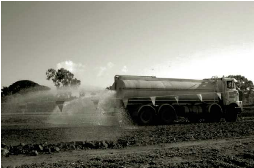
Figure 6.21 Spraying of water on each lift of soil before compaction in the field (Courtesy of N. Sivakugan, James Cook University, Australia)
