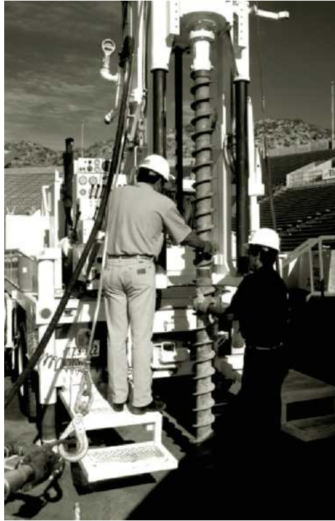
Figure 17.2 Drilling with flight augers (Courtesy of Danny R. Anderson, PE, of Professional Service Industries, Inc., El Paso, Texas)
