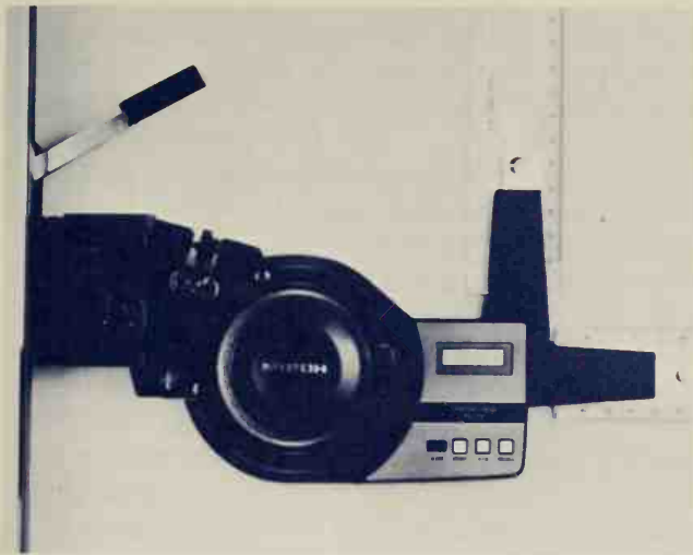
Figure 1-14 Drafting machine head with digital readout (Courtesy Consul & Mutoh, Ltd.)
