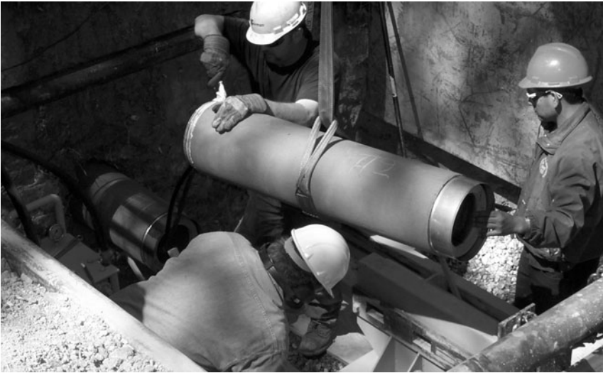
FIGURE 4-3. Vitrified clay pipe (VCP).
