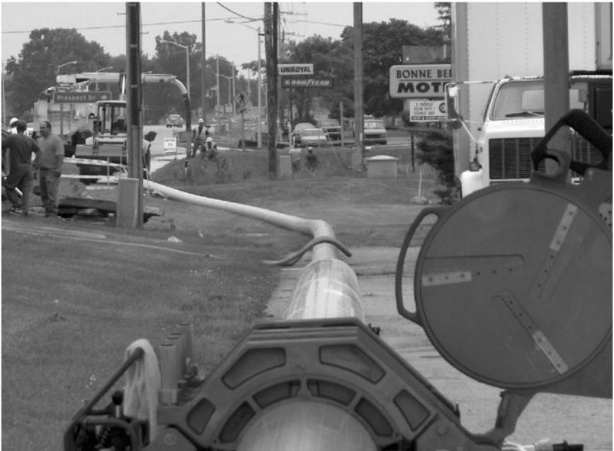
FIGURE 4-6. Pipe bursting with PVC pipe.
