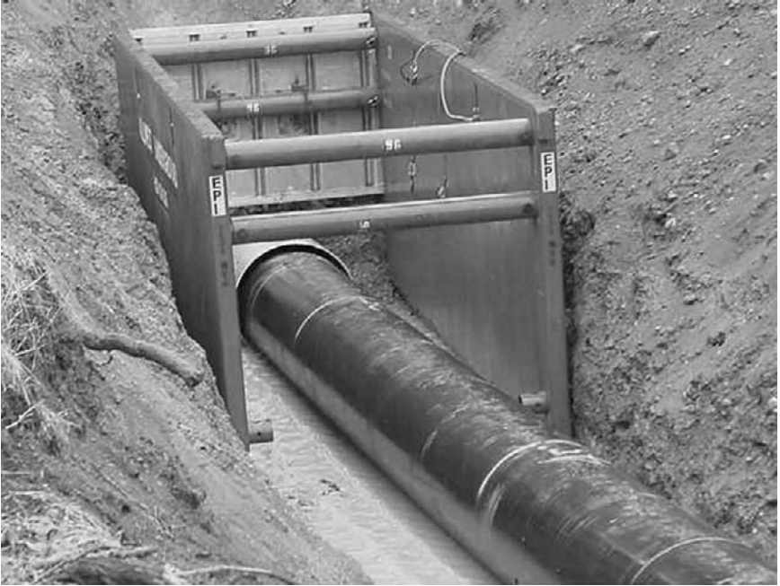
FIGURE 6-2. An example of trench shoring.
