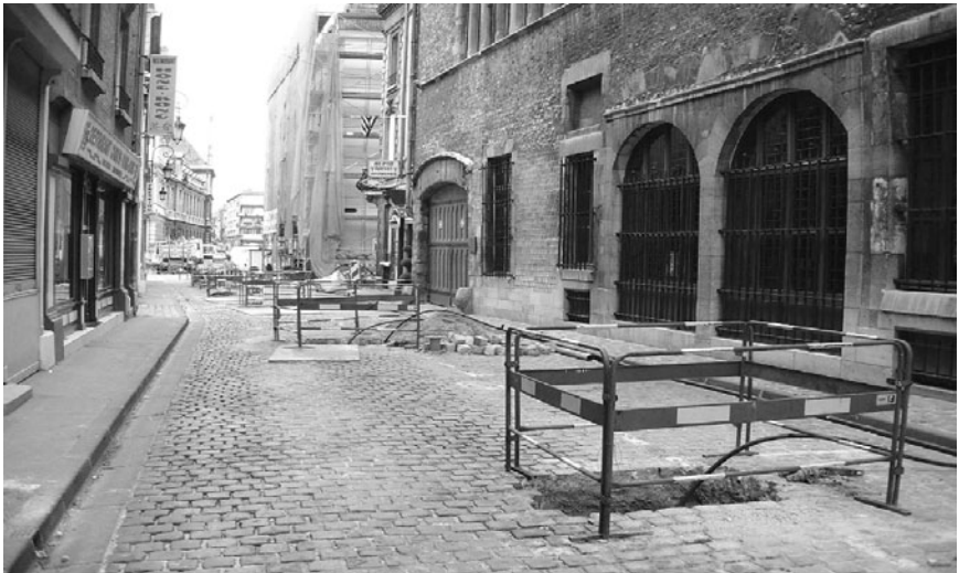
FIGURE 6-3. Service lateral excavations.
