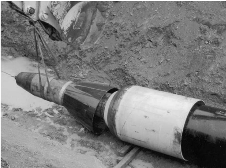
FIGURE 4-5. Pipe bursting with HDPE pipe.
