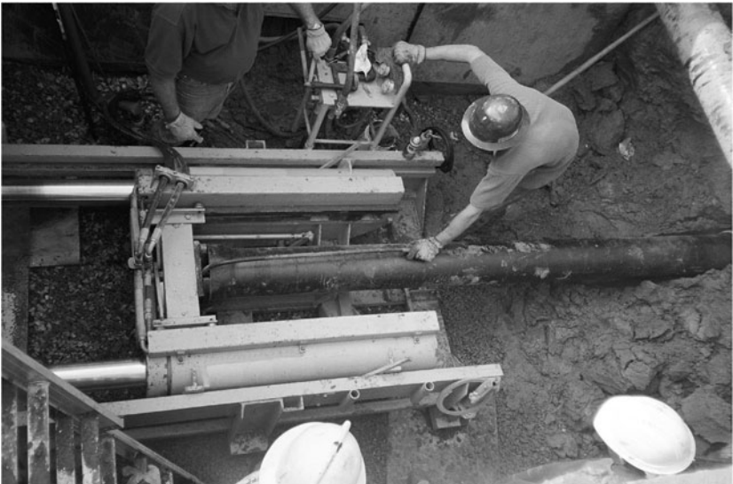
FIGURE 4-4. Pipe bursting with DIP.
