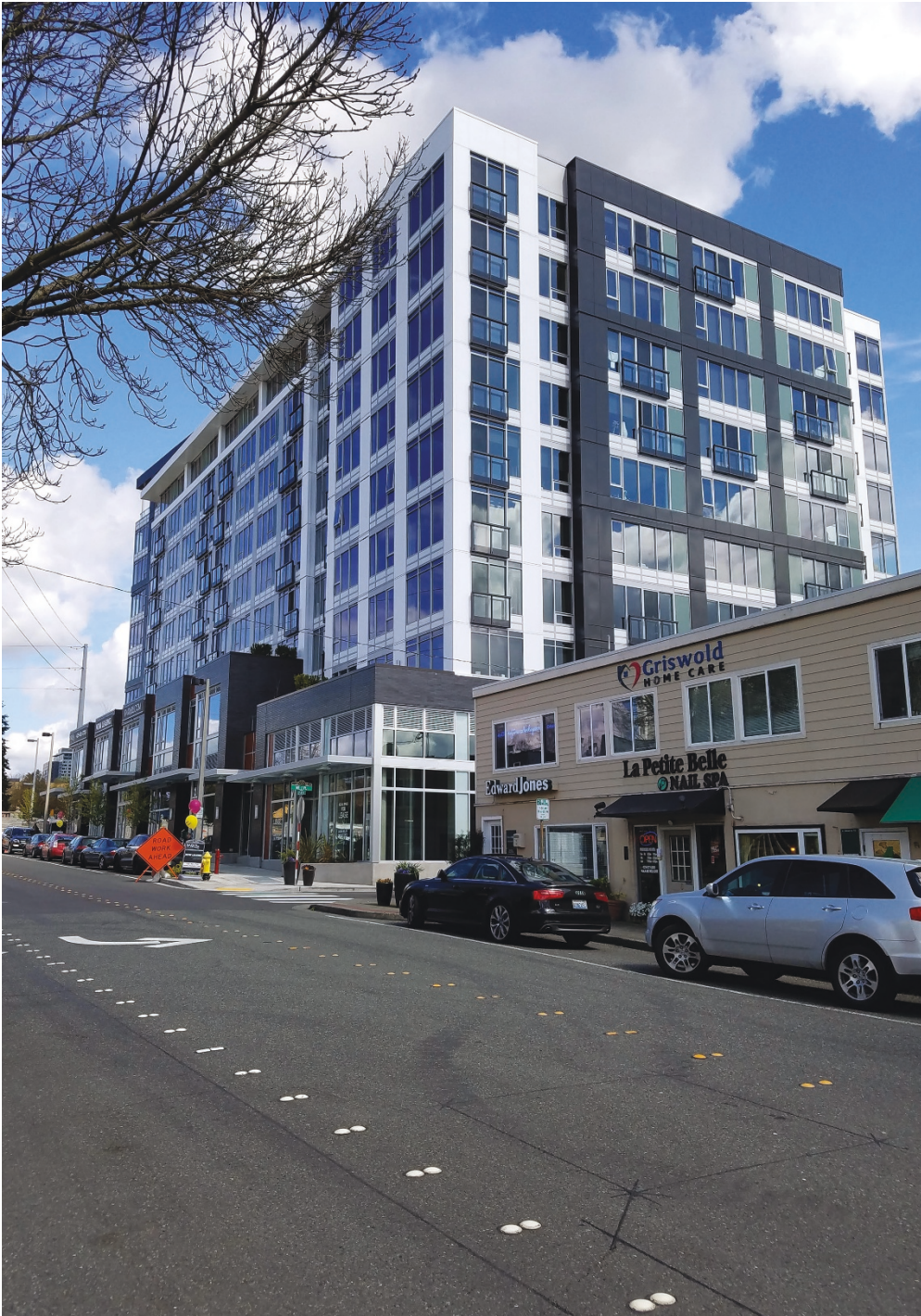
Figure 13.8. Bases of buildings reflect the scale of older existing structures. Upper floors must be set back. (Mark Hinshaw)
