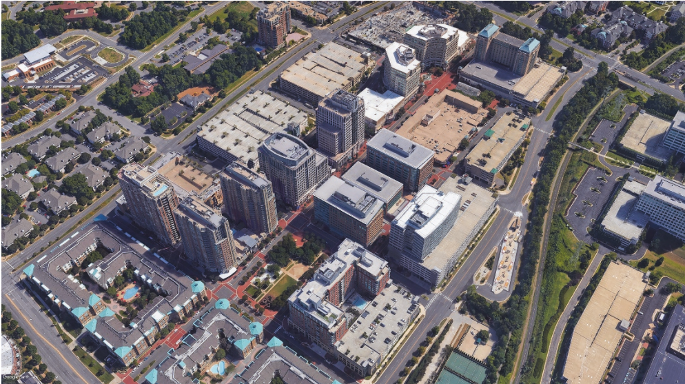
Figure 15.4. Market Street in Reston Town Center anchors a comfortable street grid that provides multiple ways to move within the center and multiple peripheral points for access to surrounding areas. (Google Earth Pro)
