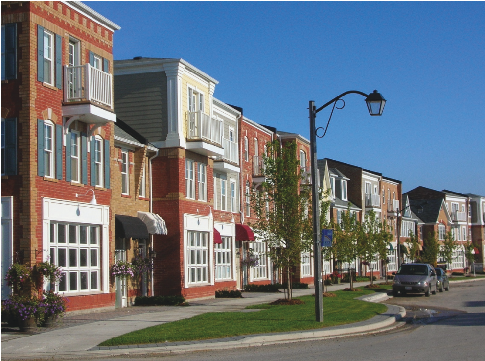
Figure 10.2. Cornell, Ontario, created a mixed-use main street with live-work housing units. (NAK Design Strategies)
