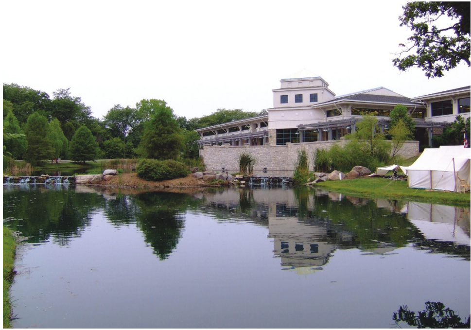
Figure 11.3a, b. Office parks generated robust fiscal benefits for Dublin because Ohio allows host communities to tax employee earnings. The result was an unusually high level of local services such as the community’s recreation center, shown below. Concerned about slowing growth in legacy office parks, Dublin adopted a plan in 2007 that proposed denser, walkable, mixed-use developments in some areas as a way of restoring employment and revenue growth. (Chart: Stantec. Photo: Wikipedia contributor Analog Kid under CC BY-SA 3.0)
