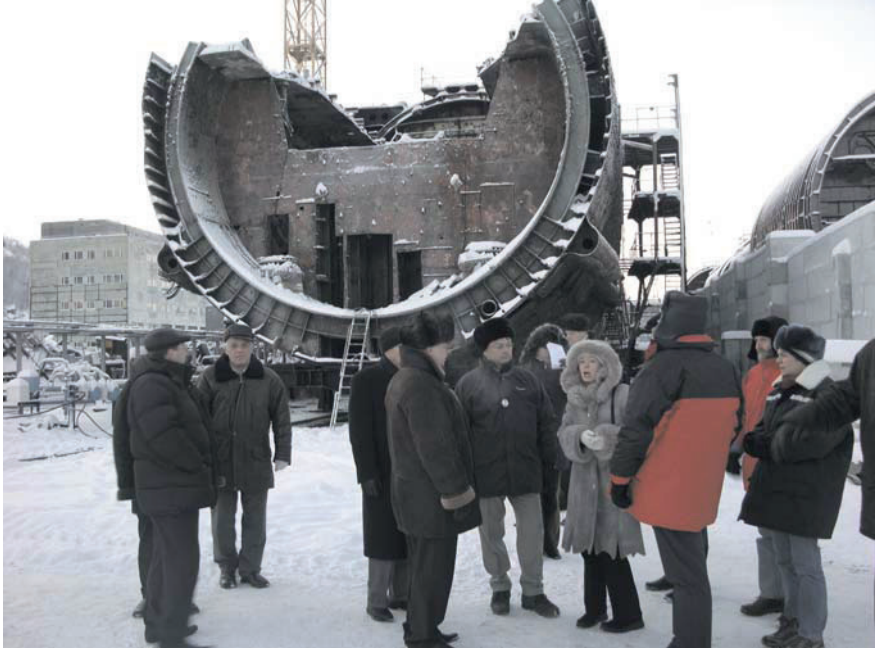
Fig. 4. Cutting reactor compartments at Nerpa shipyard (photo: Nerpa shipyard).
