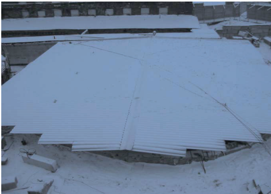
Fig. 11. A View of the new temporary, weatherproof Cover over Tank 3A
