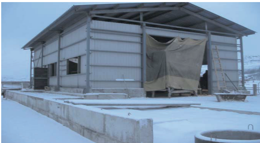
Fig. 10. A View of the partially completed, new Vehicle Decontamination Building
