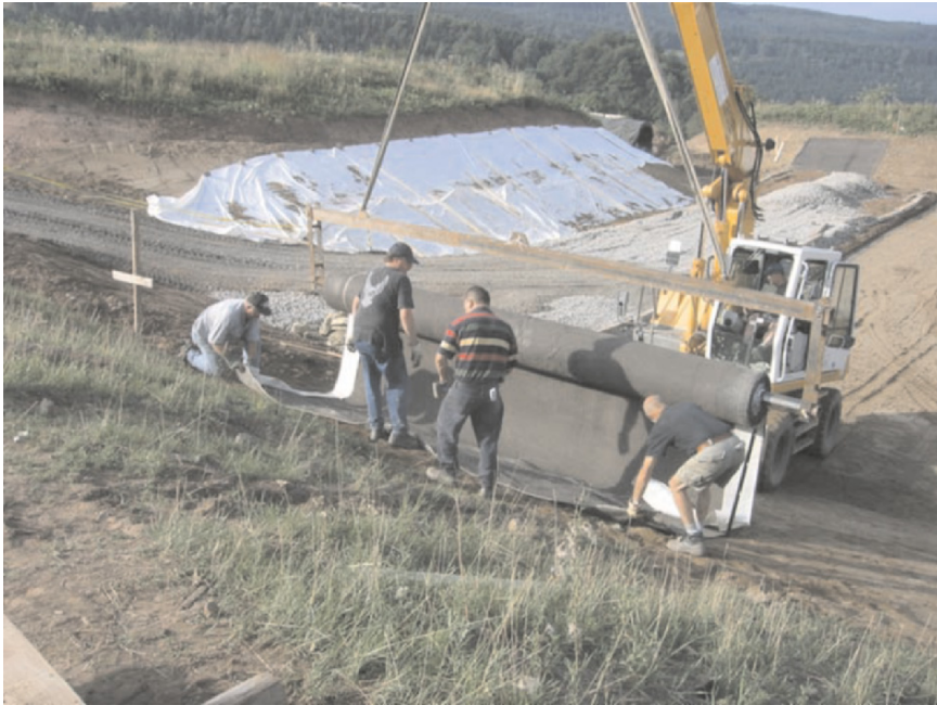
Figure 7. Laying of the Bentonit mats.
