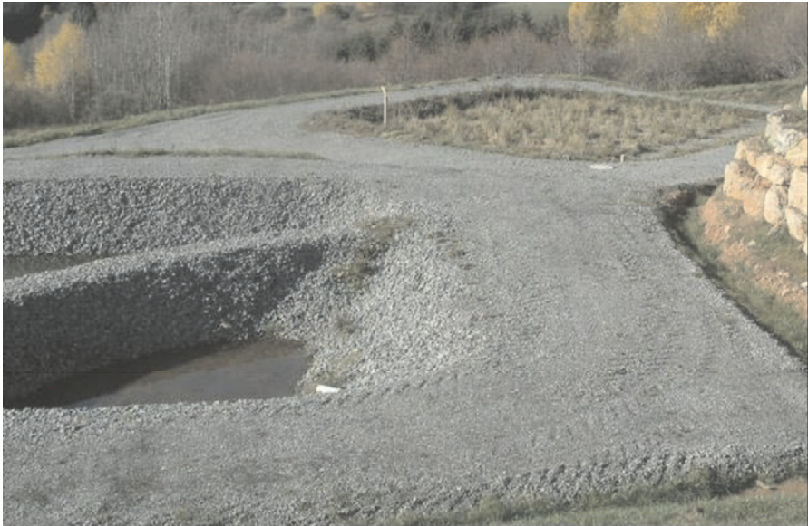
Figure 10. Treatment plant after plantation and start of operation.
