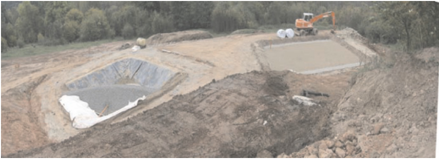
Figure 9. Placement of the inflow and outflow drainage, filling of the gravel.
