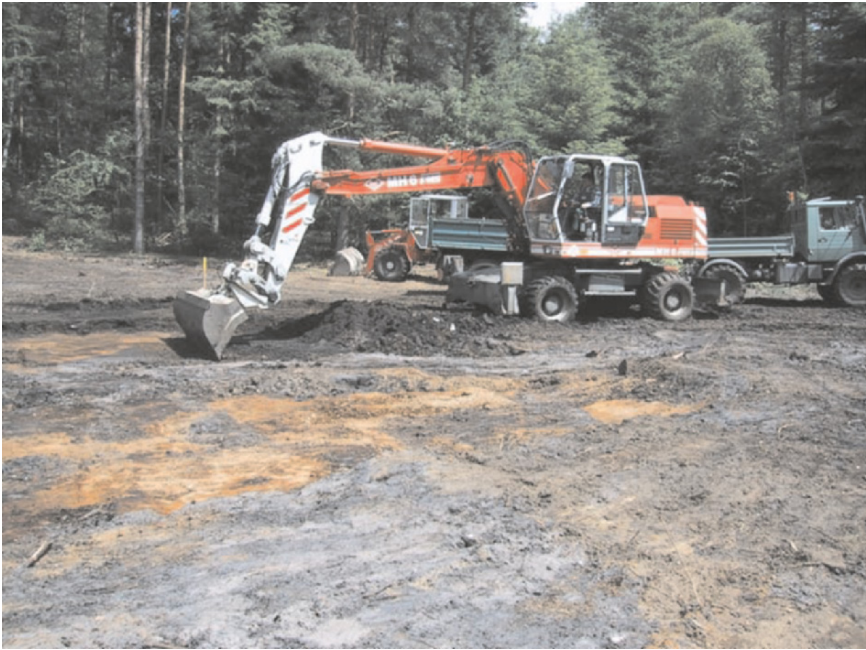
Figure 2. Excavation of the hot spots.
