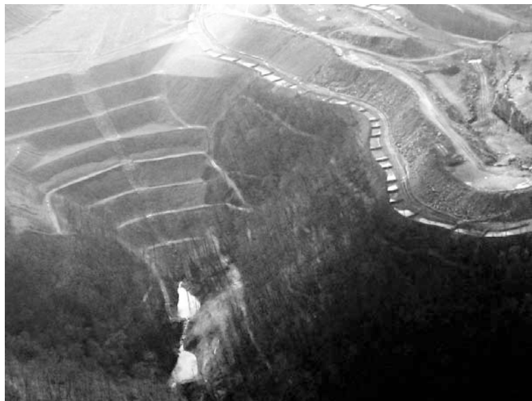
FIGURE 4.1 SEDIMENT PONDS, VALLEY FILL, AND EDGE OF COAL MINE NEAR BOB WHITE, WEST VIRGINIA, UNITED STATES.
