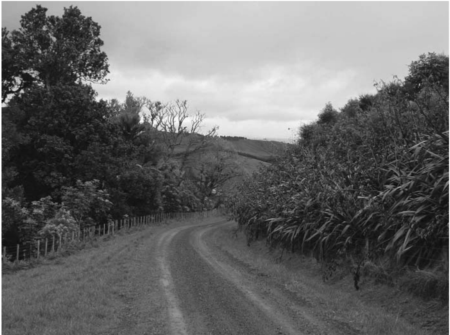
Figure 12.3 A well-formed farm track, with all-weather surface and planted up-side bank to reduce bank erosion
