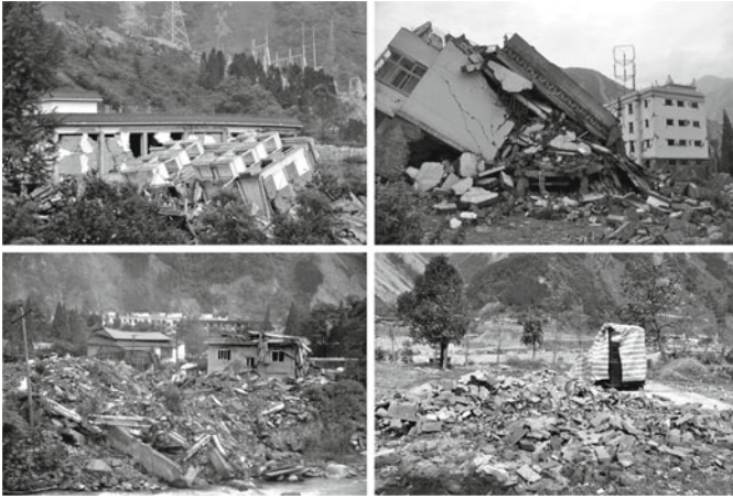
Fig. 13.2 Selected photos showing damages after the earthquake struck China's Sichuan Province. With more than 69227 casualties, this quake is cited as the worst natural disaster striking China since the Tangshan Earthquake in 1976. Photos were taken near the epicenter. Photographed by Xiaojun Yang
