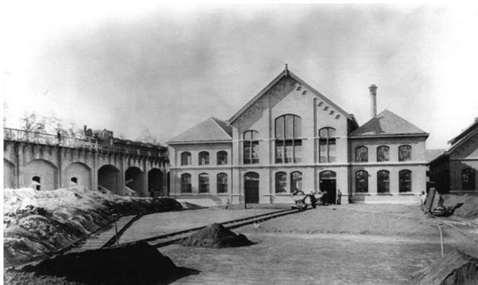
Fig. 3.2 Gas purification building of the former gasworks in Rotterdam Kralingen (built between 1884 and 1887) with iron bearing soils (“bog ore”), used for trapping of cyanide in raw coal gas, laying outside for regeneration
