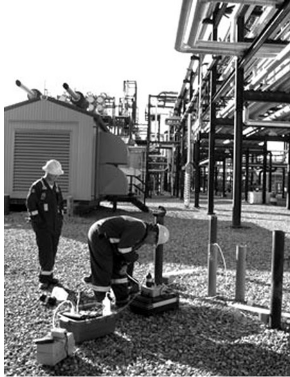
Fig. 17.6 An example of a groundwater sampling activity at an industrial site in Alberta, Canada (photo: courtesy of Alberta Innovates – Technology Futures; reproduced with permission)
