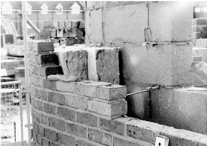
Figure 11.16 Super insulation and heavyweight internal blockwork.
