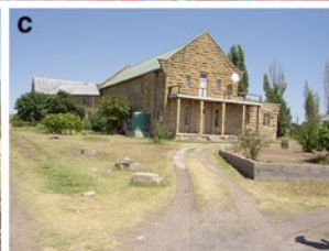
Mazenod Conference Centre/building
