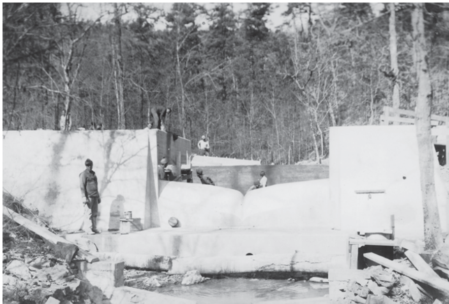
Fig. 15.4 Columbus deep notch weir ca. 1936 built by WPA and CCC labor and used to measure streamflow in Irons Fork Experimental Forest
