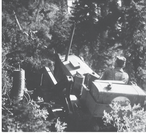
Fig. 16.1 Building a road in Deception Creek Experimental Forest in the 1930s. (From photo collection of R.T. Graham)
