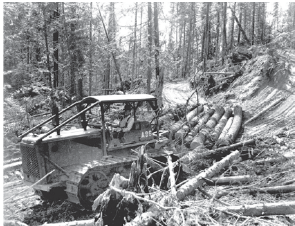
Fig. 16.5 Tractor skidders had much higher capacity than horse logging but caused increased watershed disturbance. (Potlatch Corporation: Historical Photographs © 1999)
