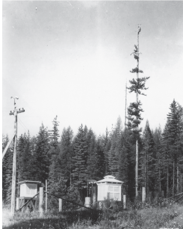
Fig. 21.7 The control weather station and George Jemison atop the 46-m western larch tree where weather instruments were maintained at the Priest River Experimental Forest in 1932
