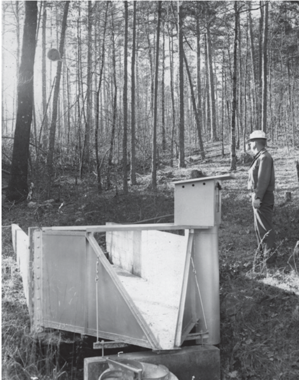
Fig. 15.5 Monitoring installation used to measure streamflow amount and collect water samples on Watershed 2 in the Alum Creek Experimental Forest. The H-flume (device with triangular opening in lower center ) is used to measure the depth of water, which can then be mathematically converted into the streamflow rate (volume per unit time). A Coshocton wheel (device offset from flume outlet) is used to capture 1% of the streamflow, which is stored in a container for later analysis. Similar installations were used at sites in Koen Experimental Forest and Battiest research area. Photograph was taken prior to the upstream basin being cut and shows typical conditions after 40+ yr of fire suppression: high density of overstory trees and thick shrub and understory growth
