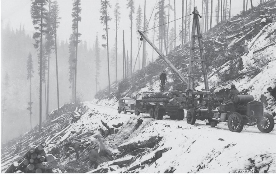
Fig. 16.3 An “Idaho jammer” cable yarder at work in Deception Creek Experimental Forest, December 1935. (From photo collections of D. Ferguson and R.T. Graham)
