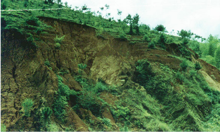
Photo 1.4 This area without good vegetation cover suffered from a landslide in Taihe prefecture, Jiangxi Province, China
