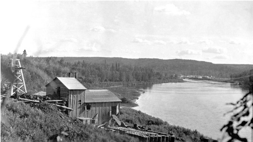
Fig. 3.14 PAA 11223 oil extraction plant – Clearwater River plant ca. 1930 appears courtesy of the Provincial Archives of Alberta. The plant processed 800 tons of oil sands in the summer of 1930, and yielded over 75 tons of bitumen (Ferguson 1985:54)
