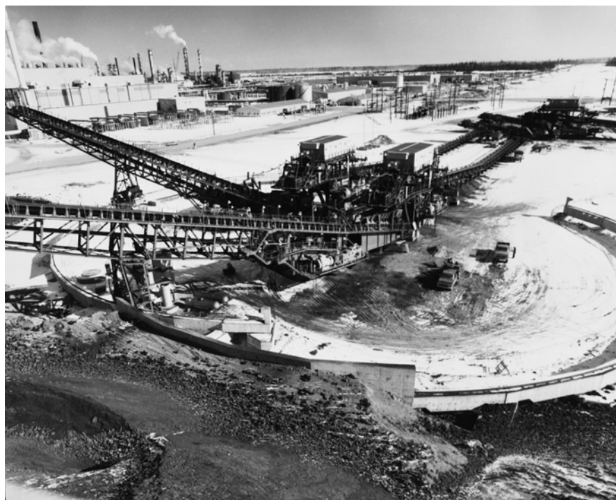
Fig. 4.4 Glenbow Archives. NA-5059-6. Syncrude plant, Fort McMurray area, AB.[ca. late 1970s]
