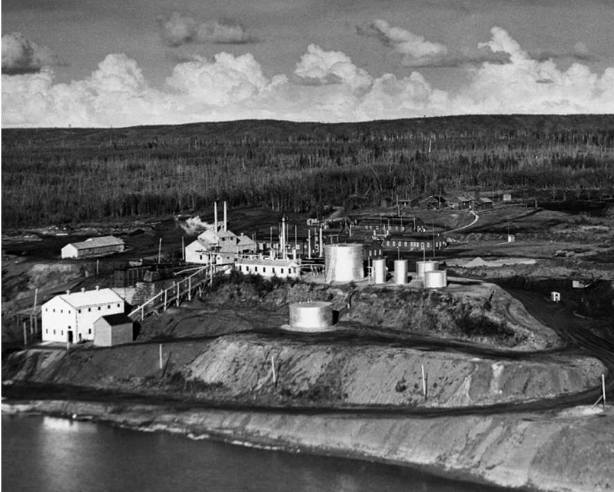
Fig. 3.20 Glenbow Archives. PA-1599-451-2 aerial view of provincial government’s pilot plant for extracting oil from northern Alberta tar sands. Bitumont, Alberta C, 1949–1950. In 1974, the Bitumont site, located 89 km north of Fort McMurray, was designated an Alberta historical site. See the statement of historic significance at http://www.historicplaces.ca/en/rep-reg/place-lieu.aspx?id=4998
