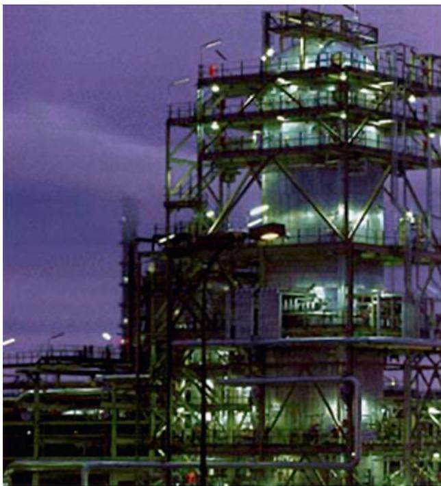
**Figure 2.3** The Fischer–Tropsch process (here showing a plant reactor at Sasol) can produce a high quality diesel fuel from biomass. The fuel is competitive if oil is above \$40 a barrel. Currently, at least three projects (Ohio River Clean Fuels, Illinois Clean Fuels, and Rentech Natchez) are combining coal and biomass feedstocks, creating hybrid-feedstock synthetic fuels. (Reproduced with the permission of Sasol Corporation, South Africa).
