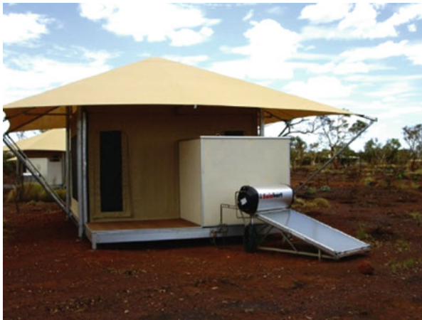
Fig. 6 Al Qurm Eco Adventure campsites—use of solar hot water. (© 2012 Eco Structures Australia)
