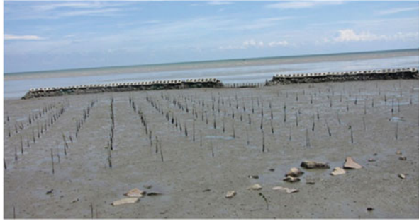
Fig. 3 L-Blocks established in study site at Sg Hj Dorani, Selangor
