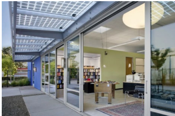
Fig. 21 Precast construction featuring integrated solar electric photovoltaics as shading device. (© 2012 Pangaeon Middle East North Africa)
