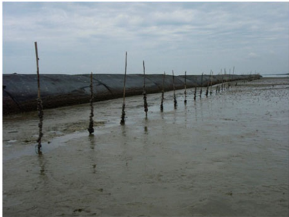
Fig. 4 Geotubes established in study site Sg Hj Dorani, Selangor
