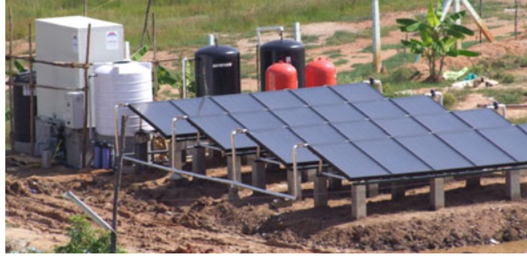
Fig. 17 Solar desalination plant produces 500 liters potable water per day. (© 1999–2013 Middle East Desalination Research Center)
