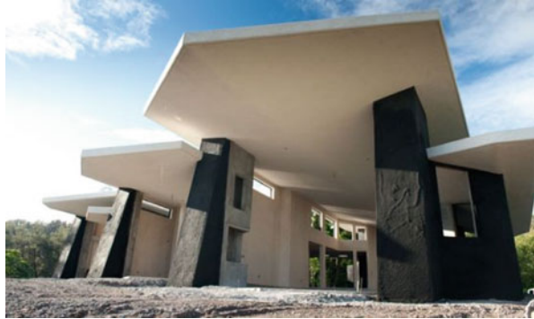
Fig. 25 Flat, expansive roof design allows for abundant shading and surface area for solar panels. (© 2012 Pangaeon Middle East North Africa)
