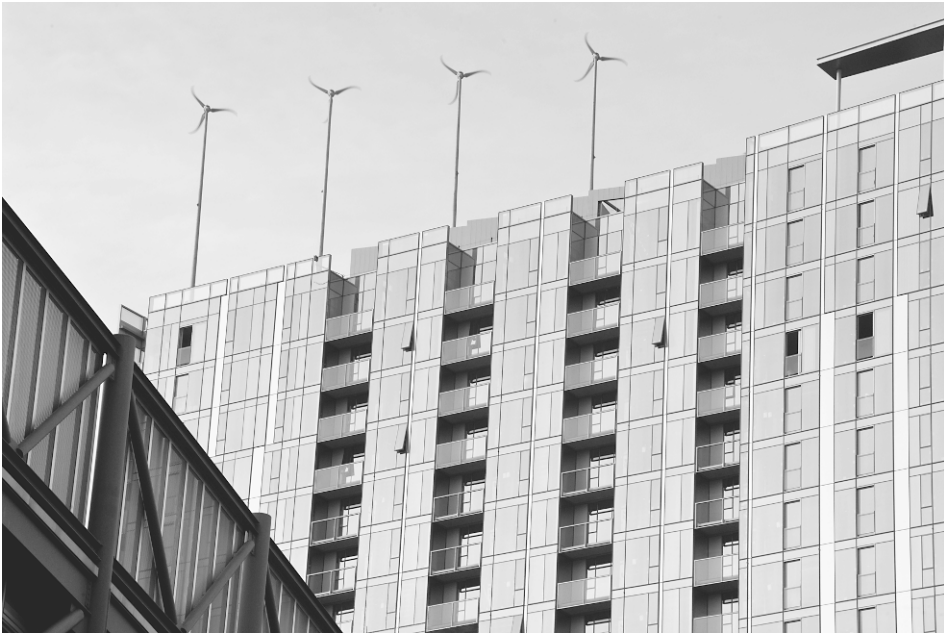
FIGURE 2.2. The wind turbines atop Indigo @ Twelve West, developed by Gerding-Edlen Development, Inc., will generate 9,000 kilowatt hours of electricity annually.
