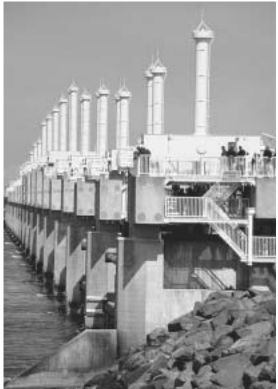
A large flood control dike in Zeeland, the Netherlands, stands ready to hold back a surging sea. © Dave Bartruff/Corbis. Reproduced by permission.
