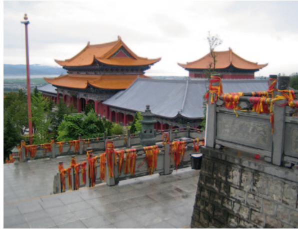
Fig. 19.1 Chongsheng temple site; eastern slopes of Cangshan near Dali overlooking and reaching down to Erhai Lake in Yunnan province, China, 2011. (Photo Gert Gröning)
