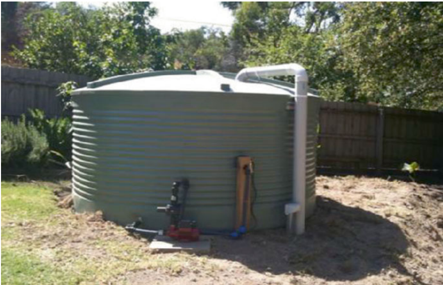
Fig. 3.2 A back yard small water storage tank
