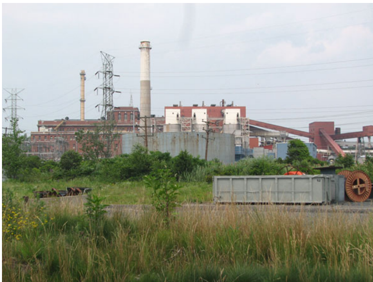
Fig. 12.3 The mid-Connecticut resource recovery facility developed on the site of an existing utility plant on the banks of the Connecticut River. The facility operates continuously and can burn coal if solid waste is not available
