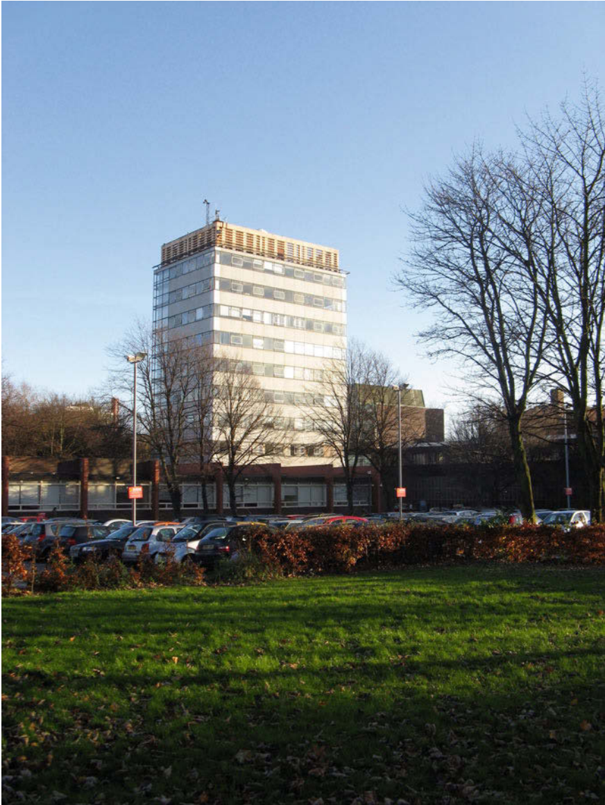
Fig. 5.17 The Chadwick Tower—the top 3 floors of which were the home of Theoretical Physics, 1959–2003: Fröhlich’s office was the right-hand half of the top floor on the side shown in the photograph, overlooking the River Mersey (Sect. 5.1)
