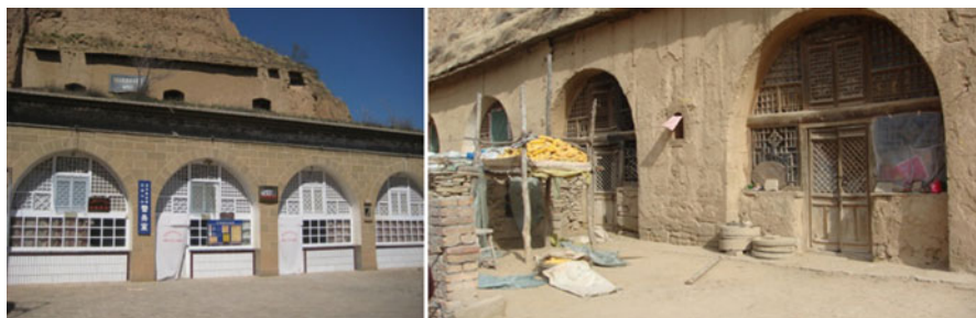
Fig. 8.6 Earth and stone cave dwellings of Gaoxigou village
