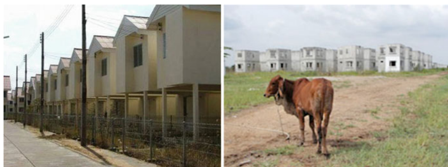
Fig. 9.3 Sample abandoned townhouse projects
