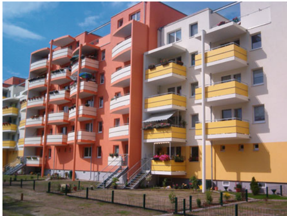
Fig. 9.2 Marzahn-Nord after reconstruction
