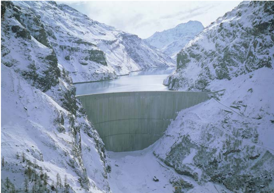
Fig. 1 The 250-m high wall is forming Lac Mauvoisin (211 Mio m 3 ) – a typical example of a reservoir in the European Alps – which contributes to the total storage capacity of about 1.3 km 3 in the Upper Rhone valley. The nominal power production for this reservoir is 350 MW. Picture: FMM SA
