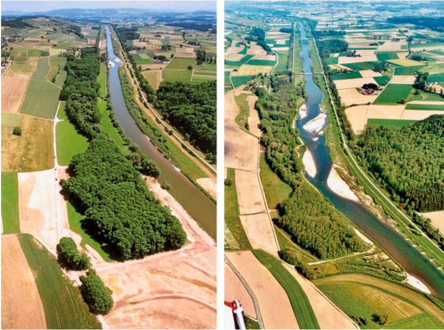
Fig. 2 The widened river bed of the River Thur at Schaffaueuli (before and after the restoration). Photo: C. Herrmann, BHA team, Frauenfeld
