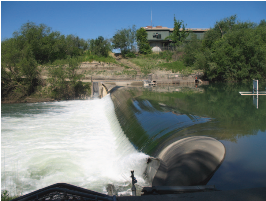
Fig. 5.11 Inflatable dam on the Russian River in California, USA is used to increase production capacity of an RBF system by increasing groundwater levels upstream of the dam and allowing surface water to be diverted from behind the dam to infiltration ponds located adjacent to collector wells. Note water diversion and pumping facilities behind the dam and fish ladders on edges of the dam to provide for fish passage
