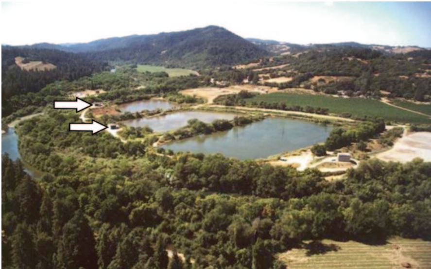
Fig. 5.12 Infiltration ponds along the Russian River, California, USA. Note location of collector well pump houses between river and infiltration ponds
