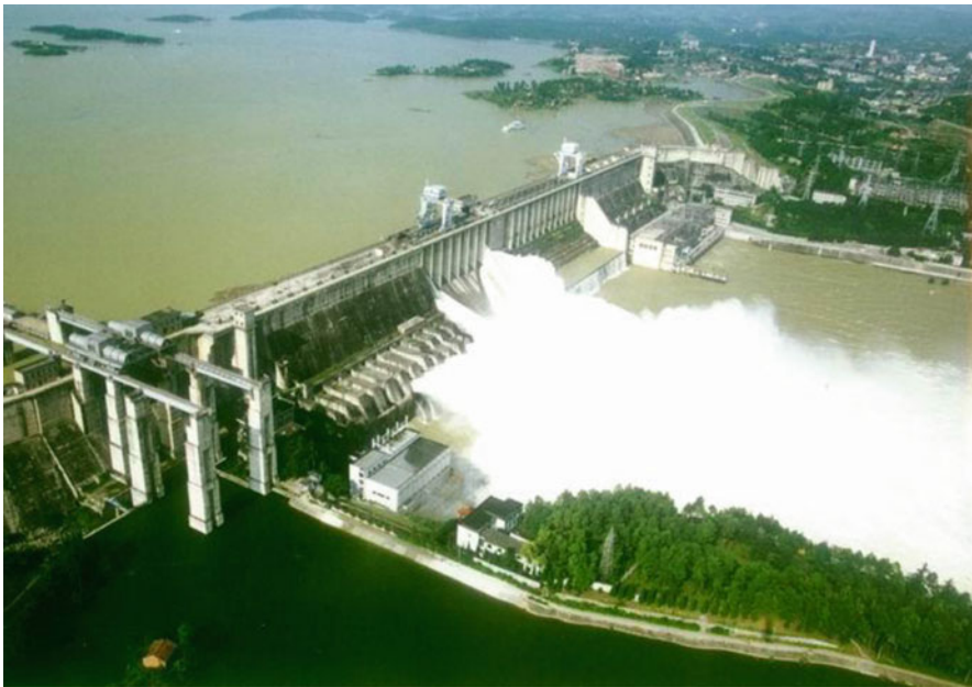
Fig. 13.1 Danjiangkou Hydraulic project
