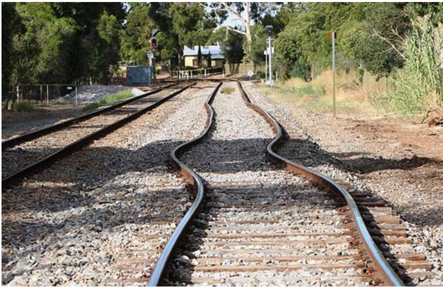
Fig. 46.11 A heat wave causing transport chaos as a result of rail line buckling (Source: http://www.worldculturepictorial.com )
