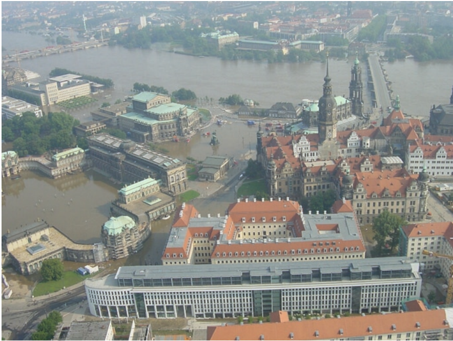
Fig. 30.3 Flood of Elbe river, August 17, 2002, water level 940 cm at gauge. Dresden, bridge Augustusbrücke (Photo: City of Dresden, Environmental office)
