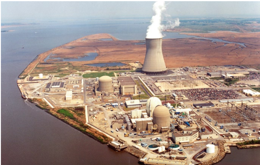
Fig. 10.3 Aerial photograph of Salem Generating Station (foreground) and Hope Creek Generating Station (background) with cooling tower
