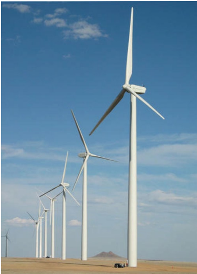
Fig. 12.1 A 2-MW wind turbine
