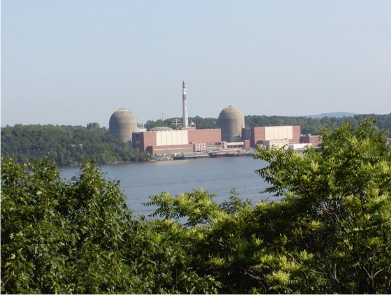
Fig. 3.3 Indian Point nuclear plant on the Hudson river (photo Michael Gochfeld)
