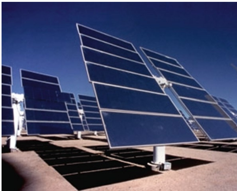
Fig. 16.1 Sun tracking heliostats at solar two, Daggett, California (Department of Energy (DOE) 1996)
