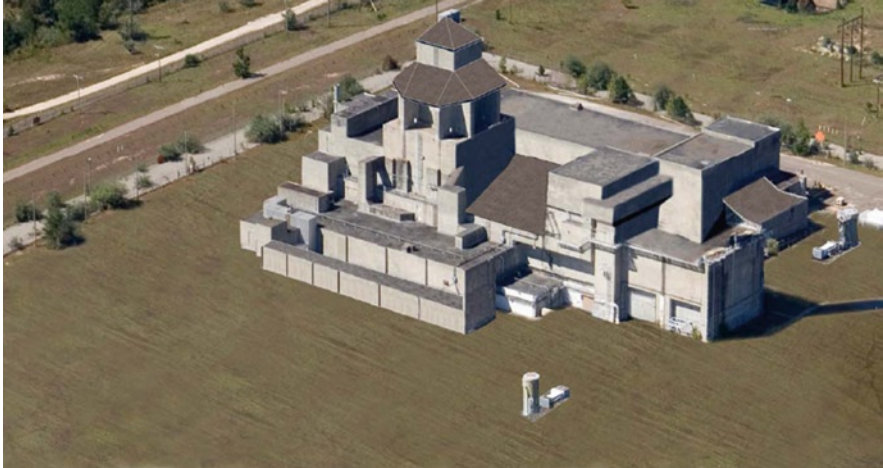
Fig. 9.7 Reactor end state for the ISD decommissioning of the P-and R-reactors at the Savannah river site (source: Hannah 2010)
