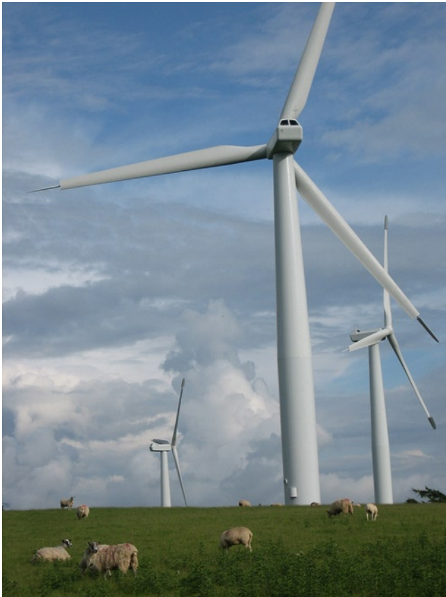
Fig. 1.3 Wind power facilities are being developed in many areas of the US, Canada, and the world, and in many places, such facilities are compatible with agriculture
