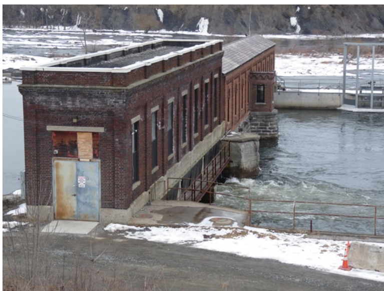
Fig. 18.4 View of the Brookfield Power Plant in Cohoes (near Albany, New York) – although this plant was established on the Mohawk River long before site neighbors or a full range of stakeholders were involved, it now solicits such participation when making new decisions
