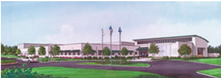
Fig. 17.1 Artist's concept of the Savannah River National Laboratory's New Center for Hydrogen Research (DOE Photo, 2004)
