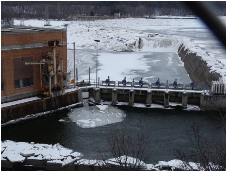
Fig. 1.2 Vischer Ferry Plant of the New York power authority, shown is the power generation plant on the Mohawk River (Schenectady, New York) at Lock 7
