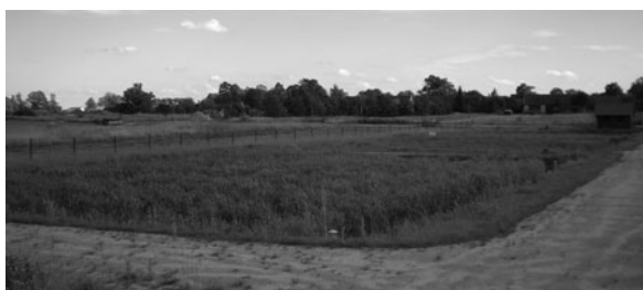
Fig. 13.3 Constructed wetland Cep, Czech Republic for 300 PE. Photo author
