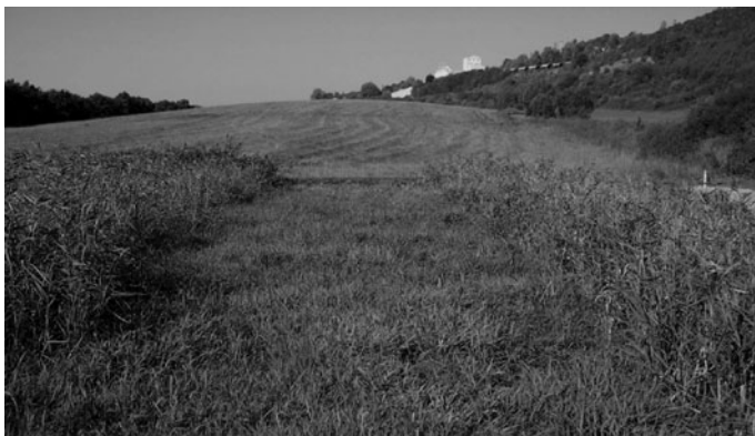
Fig. 11.2 Constructed wetland Mořina. Phalaris band in the middle, in between Phragmites bands. Photo Jan Vymazal
