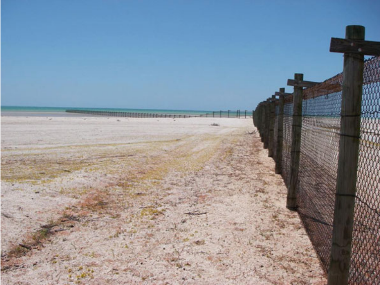
Fig. 3.3 The predator-exclusion fence at Project Eden extends into Shark Bay to minimise the possibility of introduced predator incursion at low tide. Photograph: Linda Reinhold, Western Australian Department of Environment and Conservation, Shark Bay District
