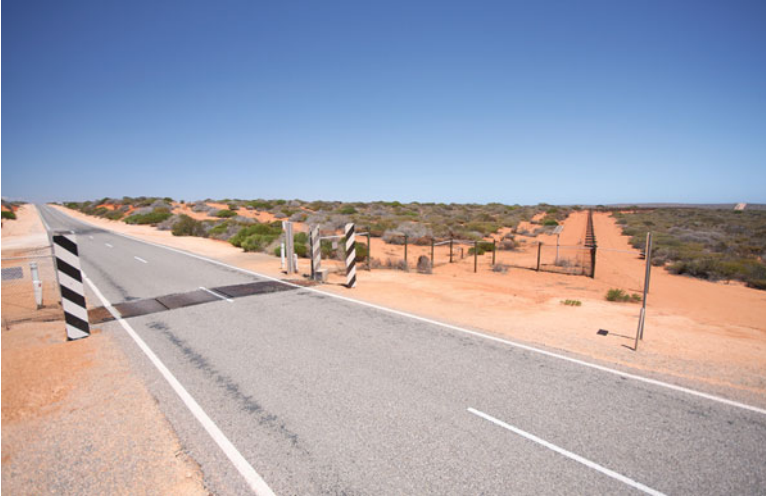
Fig. 3.2 Predator-exclusion fence at Project Eden, Peron Peninsula. The road provides public access and is a potential limitation to effective exclusion, despite the presence of a stock grid and an ultrasonic noise emitter. Photograph: Western Australian Department of Environment and Conservation, Shark Bay District
