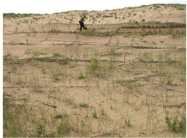
Fig. 12.8 The process of placing the straw checker-board on slopes before inoculation. Qubqi Desert, Dalateqi, Inner Mongolia, August 2008
