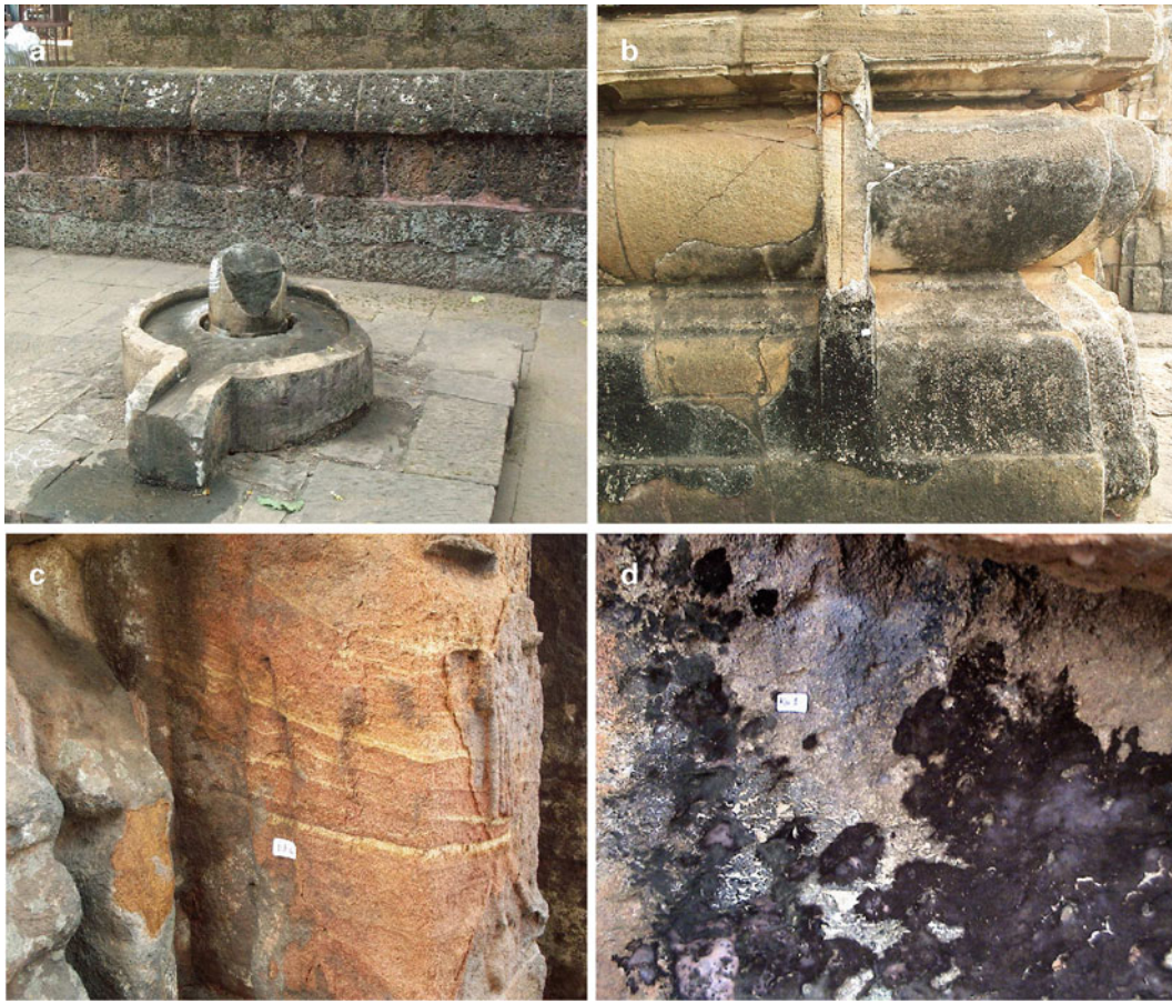
Fig. 11.4 Cyanobacterial biofilms on Hindu temples: (a, b) Abundant development of biofilms on the walls during the monsoon period leads to the formation of black crusts during the dry season;
