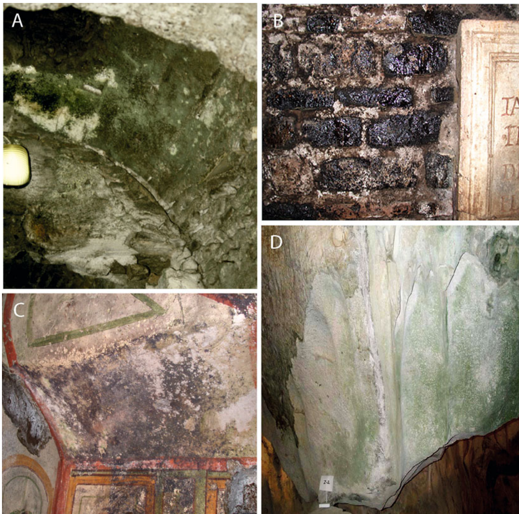
Fig. 11.6 Cyanobacterial biofilms on different lithotypes indoors: (a) Tufa rock at the Catacomb of Priscilla, Rome; (b) Brick wall in St. Domitilla catacombs, Rome; (c) Wall paintings inside the Ocean's
