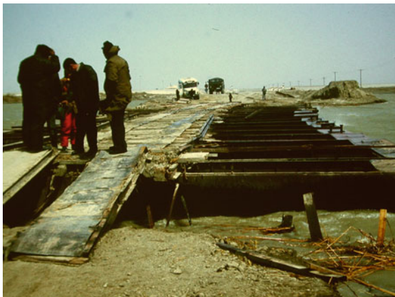
Fig. 18.14 Preliminary pontoon bridge over the Syr Darya (photo: Breckle)
