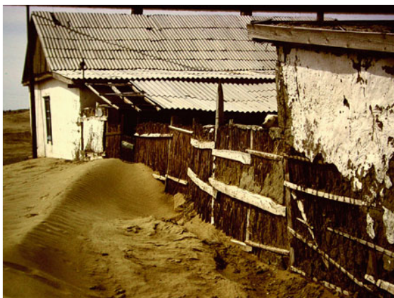
Fig. 18.7 Sand dunes cross the village of Bugun and destroy house walls by sand blasting (photo: Breckle)
