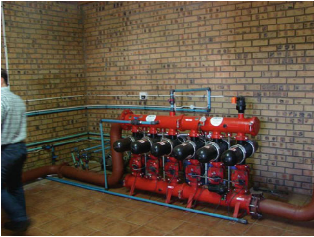
Fig. 19.5 Adequate filtration must be provided for the drip systems. This photo illustrates a manifold of sand filters from a surface water source (Photo by K. T. Morgan)
