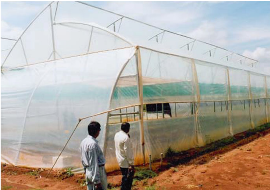
Fig. 9.6 No overlapping and fixed plastic film at the gable end
