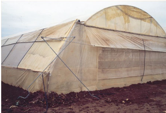
Fig. 5.18 Sloped side walls covered with insect screens and rolling-up ventilation in Jordan
