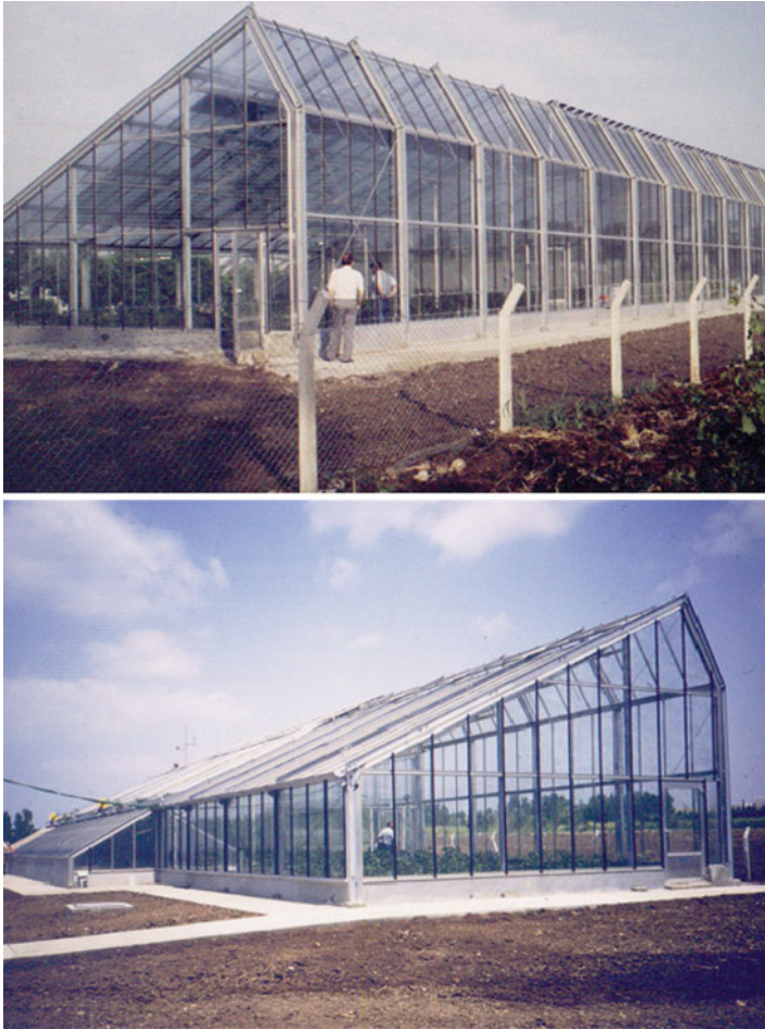
Fig. 15.11 Closed-system greenhouse type Hannover
