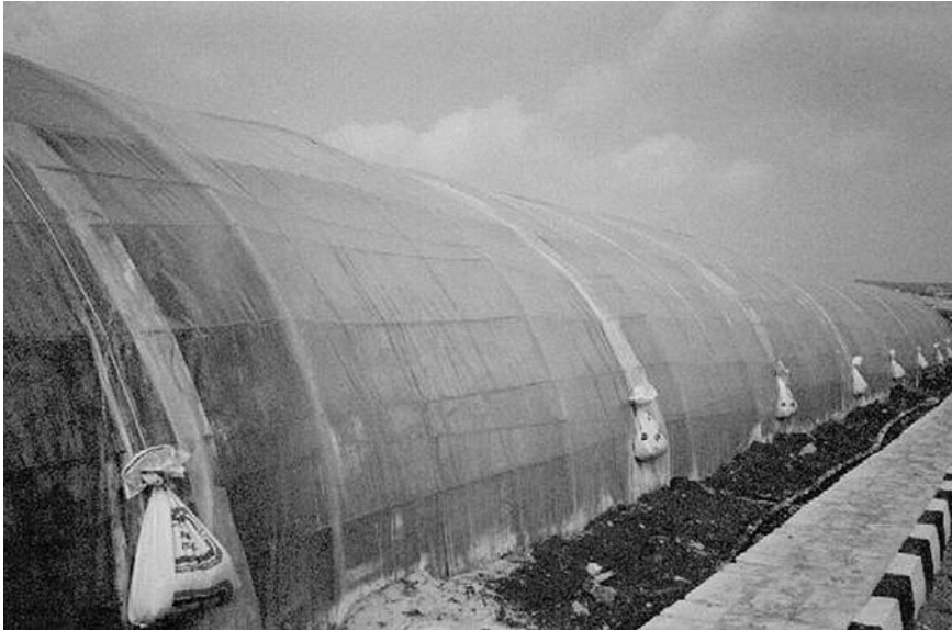
Fig. 5.8 Greenhouses without foundations are secured against uplift forces by sand sacks (Jordan). Point foundations are preferable
