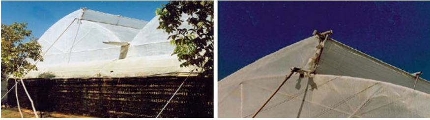
Fig. 9.15 Roll-up ventilation at the ridge of a round-arched greenhouse that has fan and pad cooling at the same time (Iran). The natural ventilation is for transit times, and has to be closed when fan and pad cooling is on
