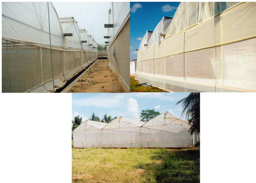
Fig. 10.14 Very well-installed and fixed insect screens at side walls and ridge ventilators
