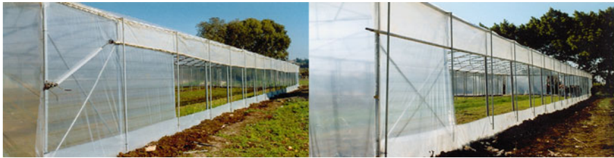
Fig. 9.4 Very well-designed roll-up ventilator with sufficient overlapping at the gable end to prevent leaks and destruction by wind forces. The horizontal roll-up tubes are nearly straight at a length of about 30 m
