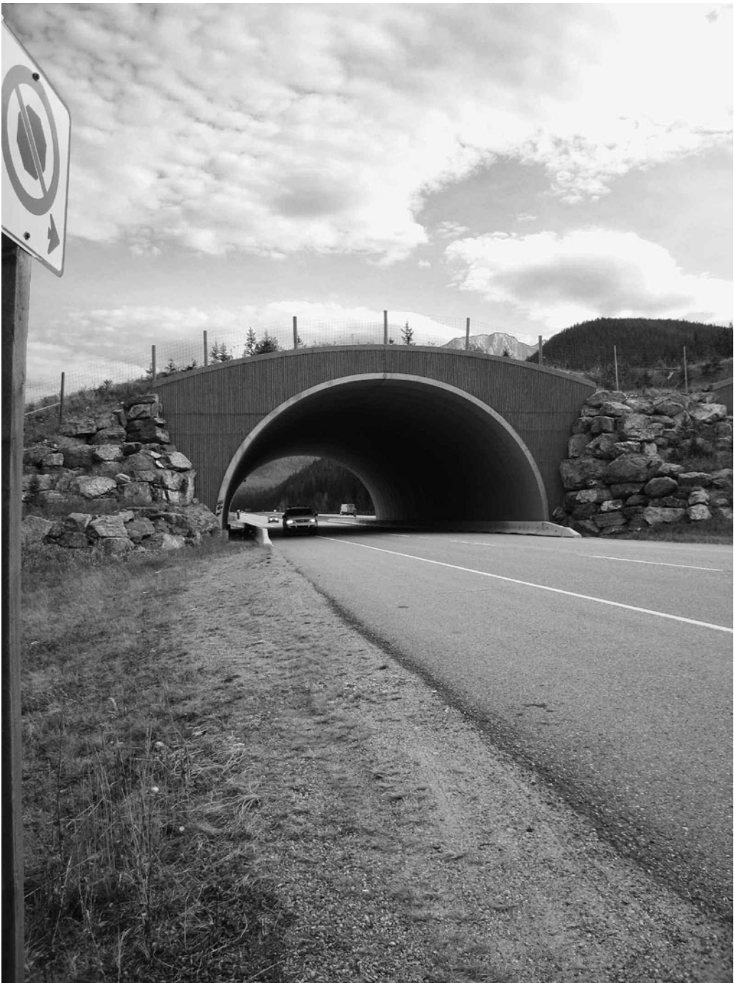
FIGURE 19.3 Across the Trans-Canada Highways bisecting Banff National Park, more than twenty-five wildlife underpasses and overpasses have been built to enhance wildlife connectivity, including this overpass. Photo courtesy of WCS Jodi Hilty.
