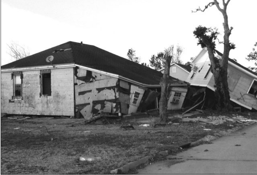
Escape route from rapidly flooding attic, as cut by butcher knife while storm waters continued to rise (see left side of roof, near the top). Photograph by Robert Gramling.
