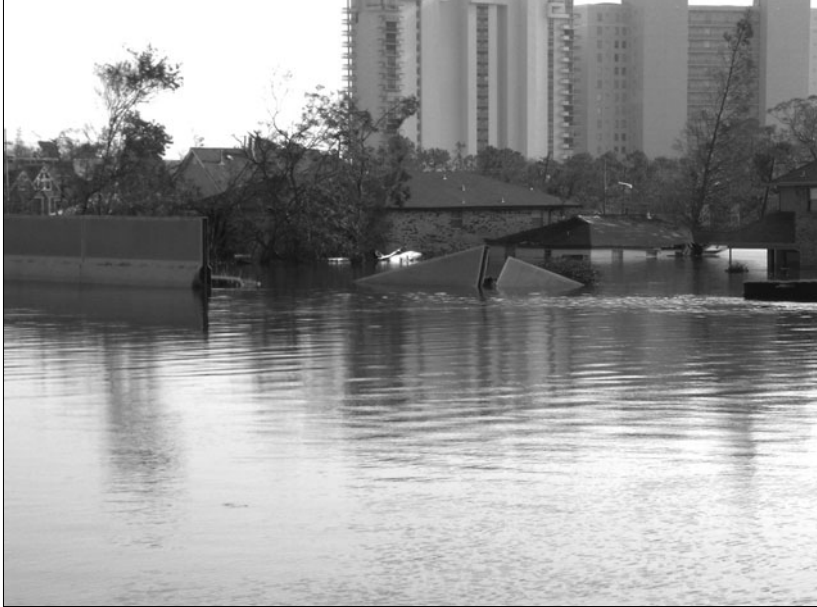
Water flowing slowly out of 17th Street Canal, August 30, 2005. Note that water levels barely reach the bottom of the concrete portions of the wall, roughly eight feet below the top of the wall. Photograph by Nathan Bassiouni.
