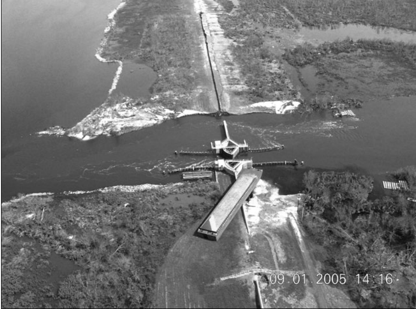
September 1, 2005, photo of Bayou Bienvenue breach, looking along MRGO Levee, toward the southeast, as used in Corps presentation to New Orleans residents. Photograph courtesy of U.S. Army Corps of Engineers, New Orleans District.
