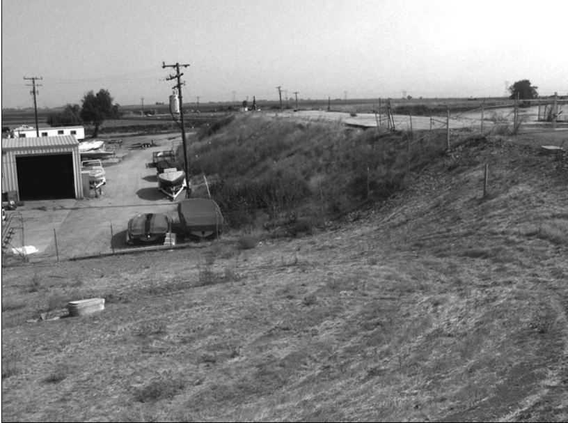
California Delta scene, fall, 2007. Note that the “Island” or land area, to the left, is well below the level of the water, on the right. Photograph by William Freudenburg.
