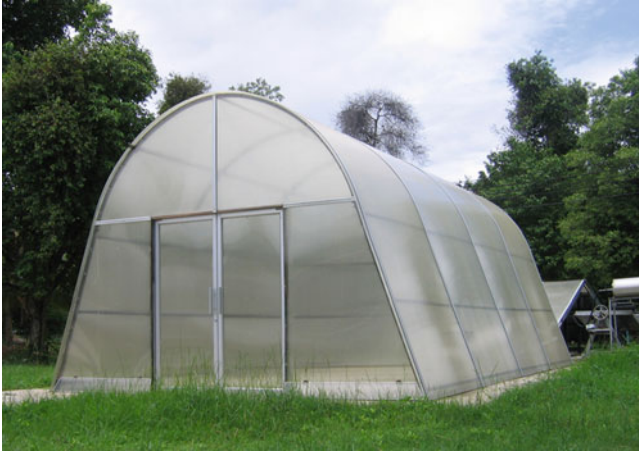
Fig. 8 Greenhouse-type solar dryer with polycarbonate sheet
