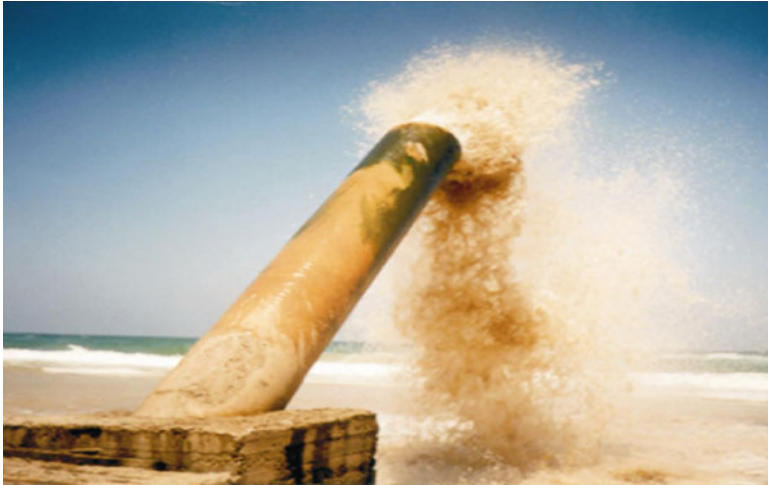
Fig. 1 Wastewater outfall along Gaza coast
