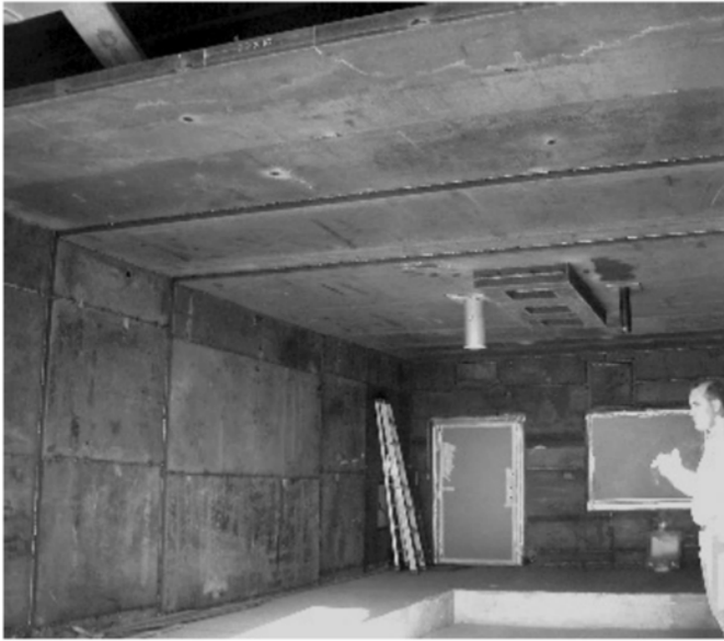
Figure 10. Shielding installation for a 9.4T/650-mm bore magnet.
