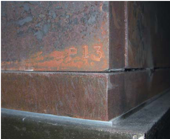
Figure 2. Electrical isolation of the iron room was ensured by isolating the iron floor from the concrete slab with a dielectric polymer paint and 10-mm thick PVC plastic sheets. The inside joints of the iron blocks were welded continuously to ensure RF integrity. The concrete slab was made independent of the surrounding building to prevent vibration transmission into the magnet room. Electrical grounding was achieved at a single point at the penetration panel and used for all electrical grounding of the scanner electronics. See attached CD for color version.
