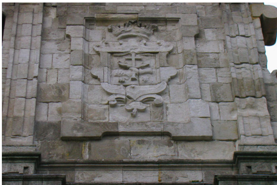
Fig. 2.4 Erosion of stone elements with marked depth and disappearance of decorative elements in granite
