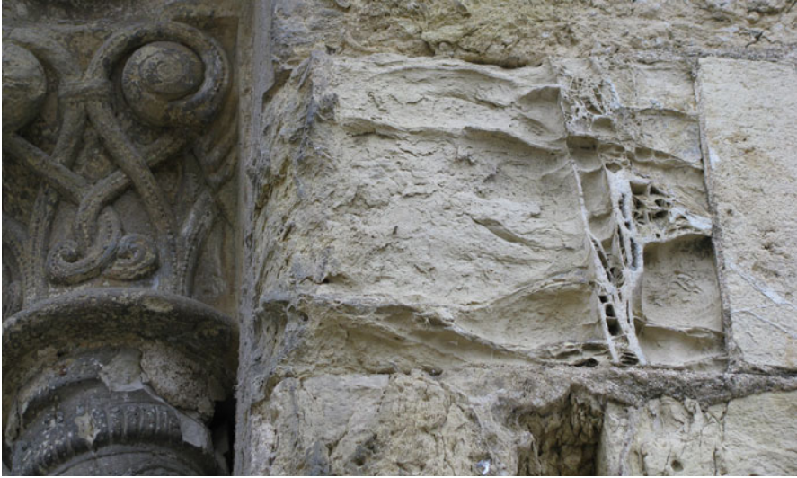
Fig. 2.1 Differential erosion in limestones associated with the presence of heterogeneities
