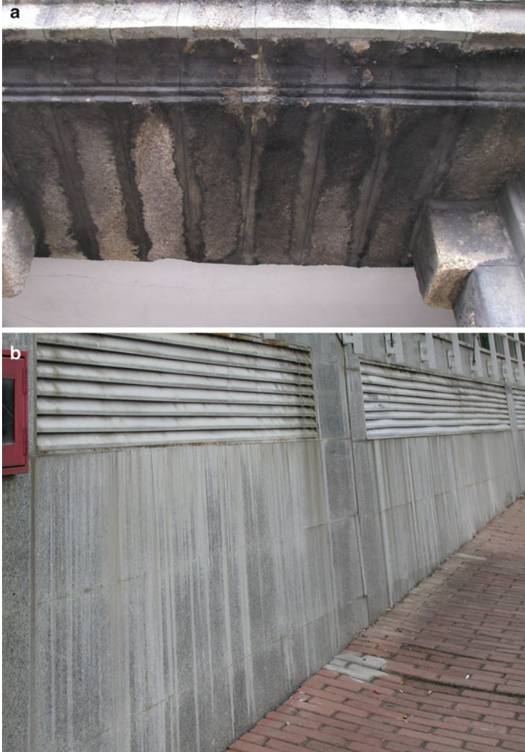
Fig. 2.2 Examples of common coatings on the built environment: (a) black crusts; (b) white crusts. Both on granitic stones
