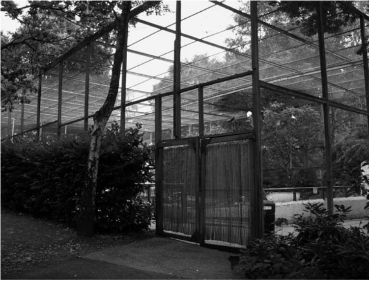
Fig. 3.3 Large flight pen with good natural screening in the form of a hedge together with screened doors which protect the birds from external disturbance (picture: Jane Cooper)
