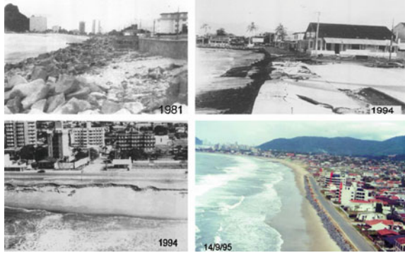
Fig. 12.8 Photos of the Shore in 1981, 1994, and 1995. Walls of concrete were applied as protective tools against the encroaching ocean. Source Angulo et al. (2000)
